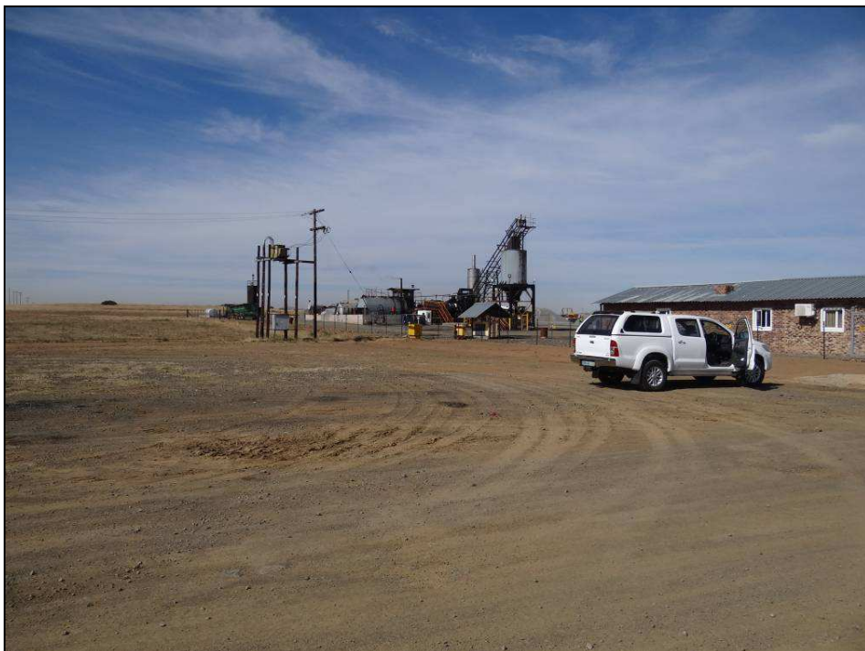
Fig.1 Point A at the proposed Supa Asphalt site facing Point B.
