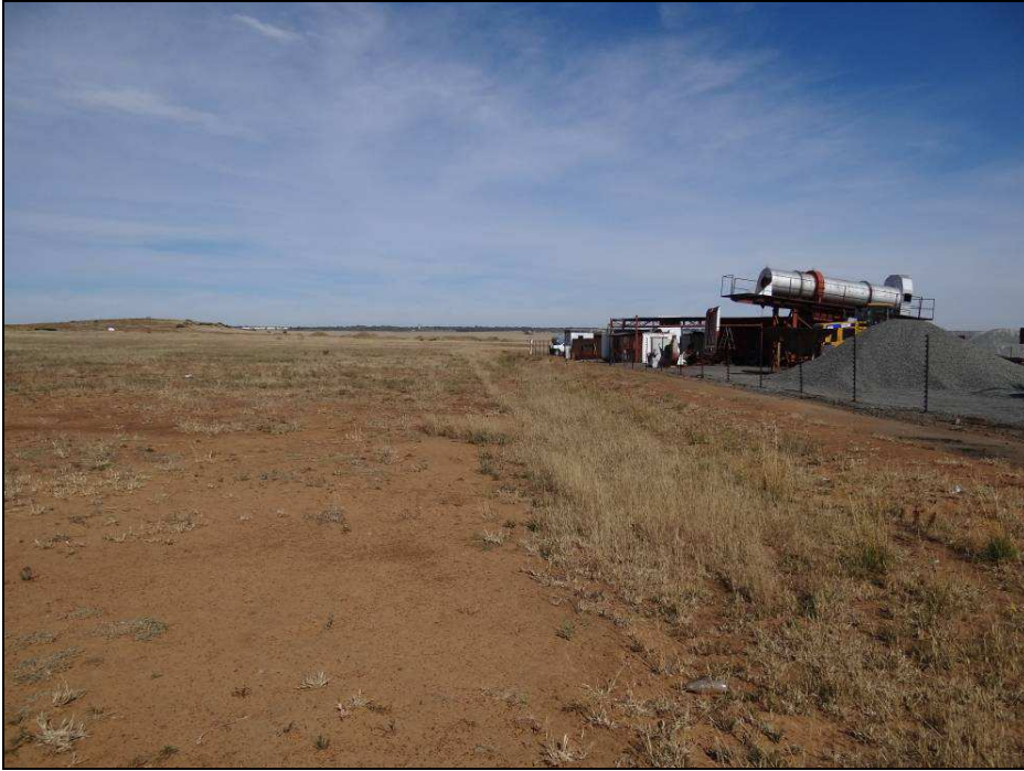
Fig.2 Point B at the Supa Asphalt site facing Point C.
