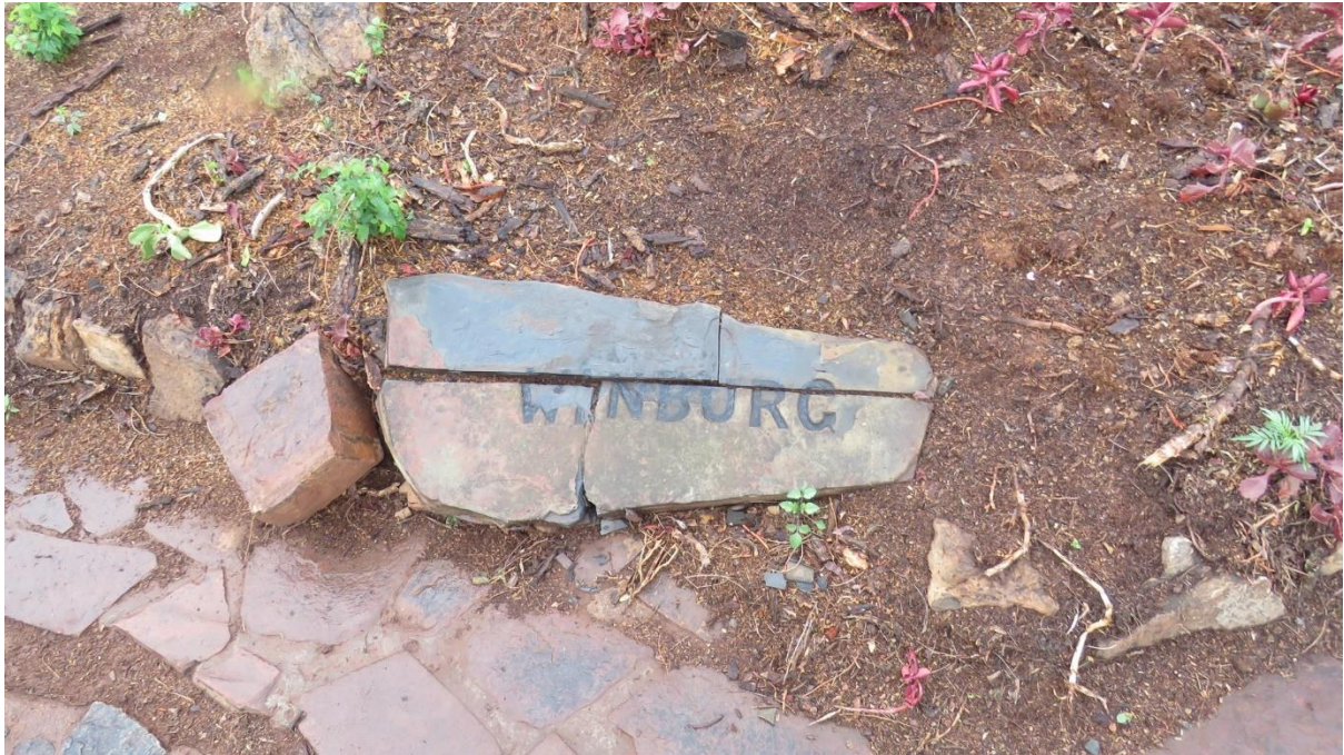
Figure 59: Example of damaged signage that will be replaced.
