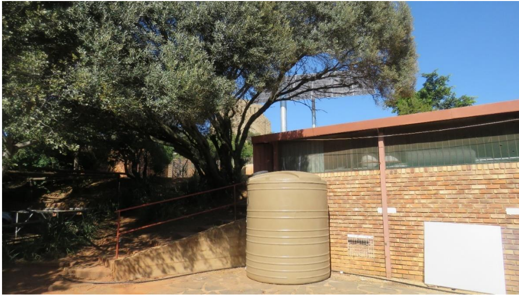
Figure 88: Building at the workshop area.
