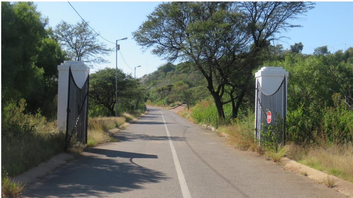
Figure 120: Former entrance gate to Fort Schanskop.
