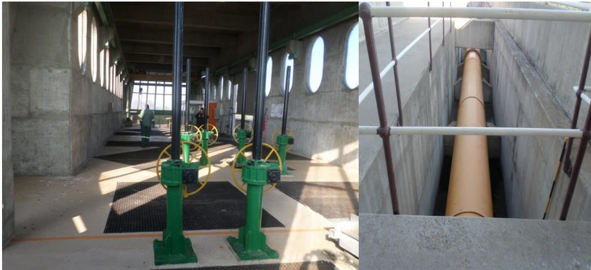
Figure 3: Start of pipeline at the Sedibeng Water Main Reservoir
