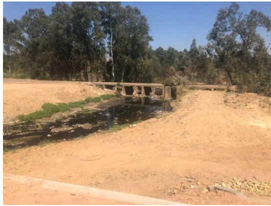
Figure 8 - View of old Crownwood road bridge
