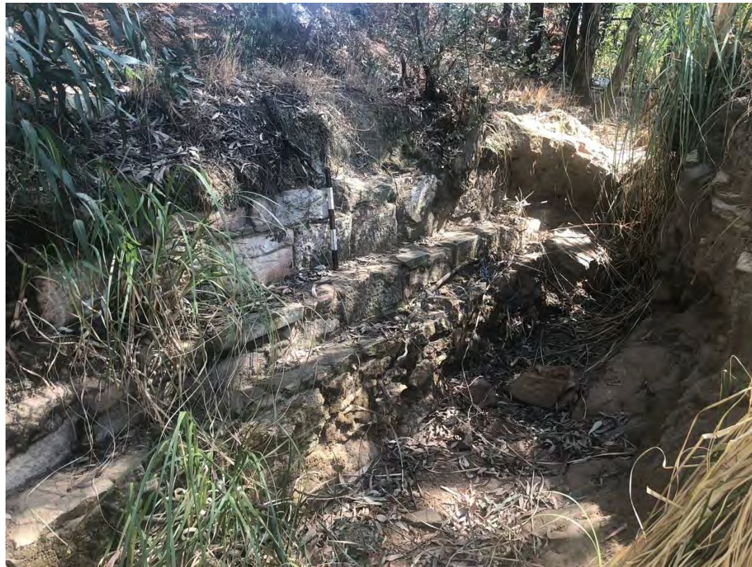
Figure 27 – Exposed stone walling at VS1
