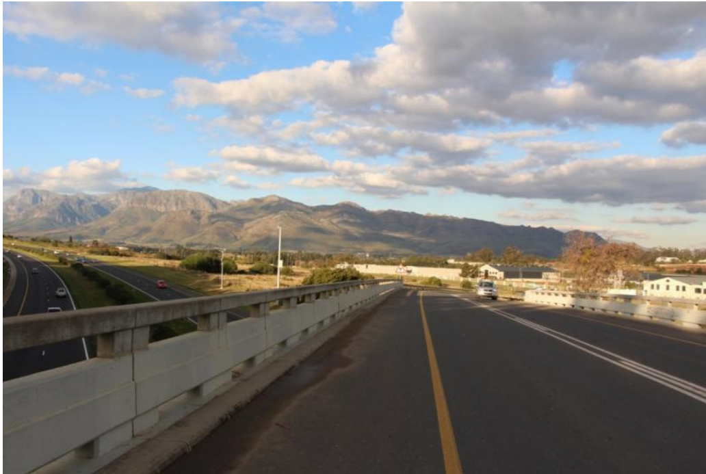
Image 18: Viewpoint 12 (from Suid-Agter-Paarl Rd bridge looking south)
