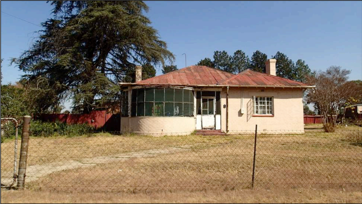
Figure 23. Type B Building showing bay window
