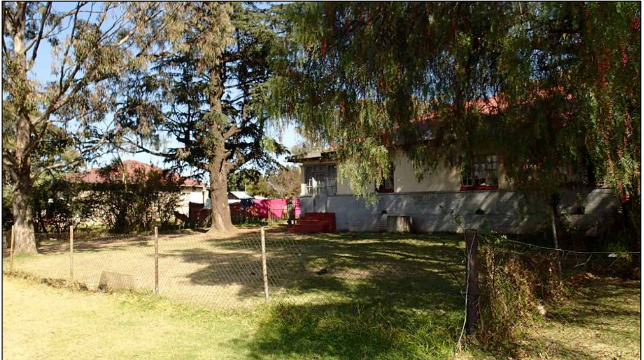
Figure 26. Type C Building
