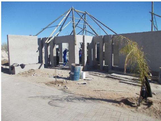
7(c) Construction on-site at the time of our study
