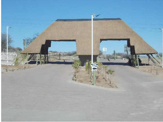
7(a) Existing thatched roof entrance to resort development
