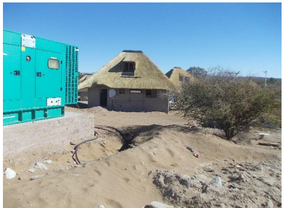
7(d) Construction on-site with a generator
