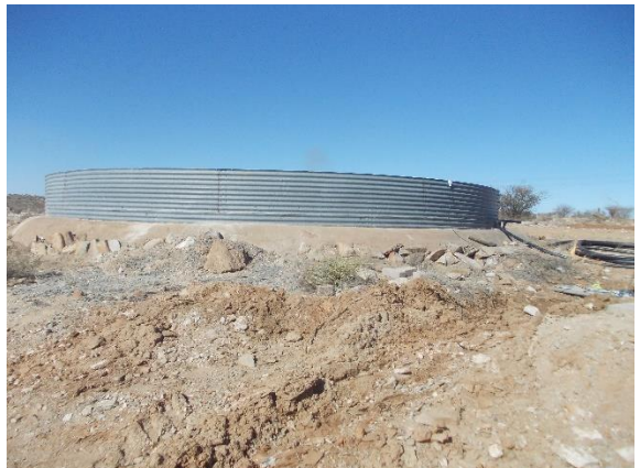
7(f) Reservoir on site adjacent to waterworks/supply
