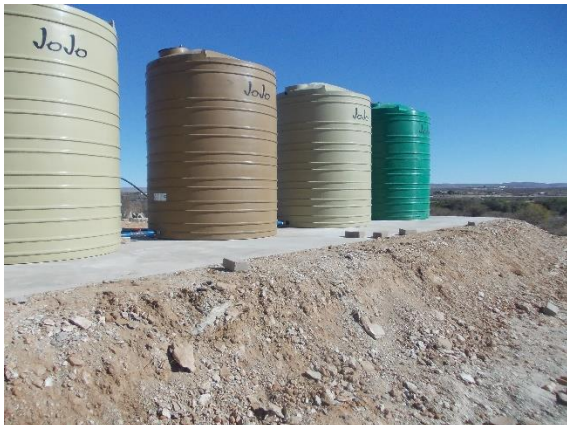
7(e) Waterworks/supply with a foundation on study area
