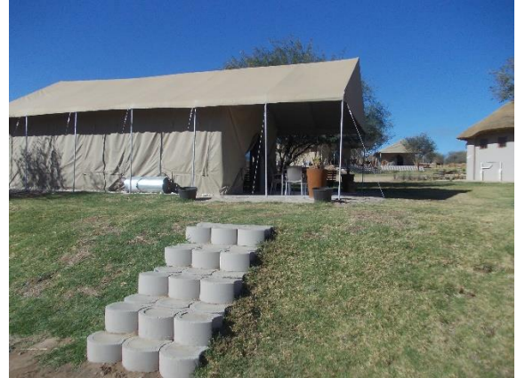
7(b) Existing tented chalets on development
