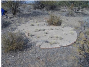
18(a) Cement foundations
