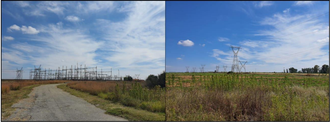
Figure 5-8: View of the western offset of the project at the Eskom substation (left) and the project corridor through cultivated land (right).
