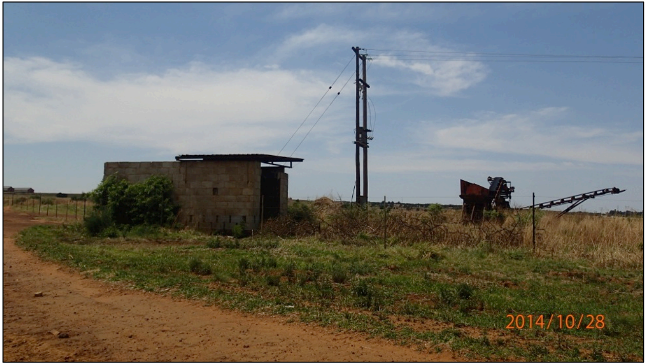
Figure 12. Pump house and crusher conveyor located within the study area
