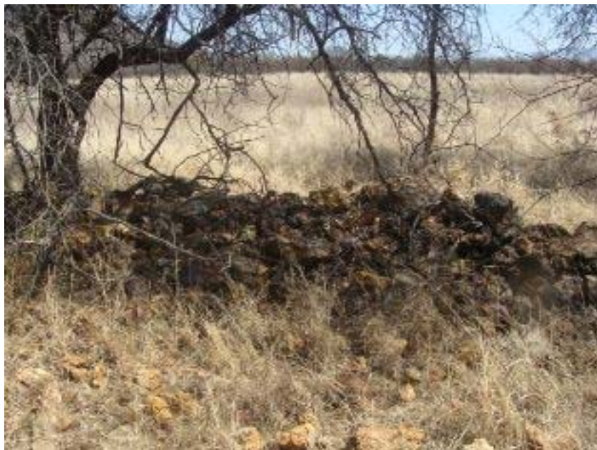
Figure 16: Foundations of stone and cement structure.
