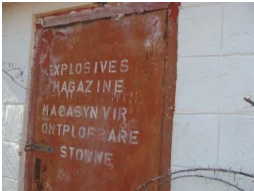
Figure 18: Close-up of explosives magazine door.
