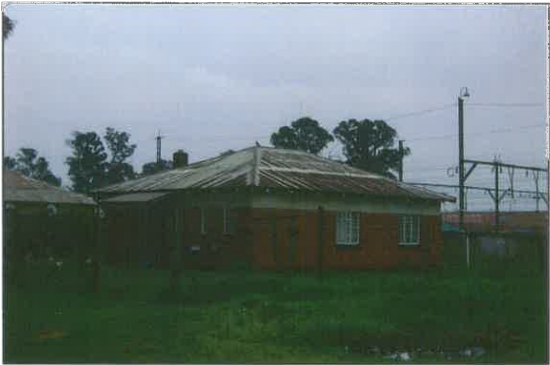
Figure 12. Typical station house at Delmas
