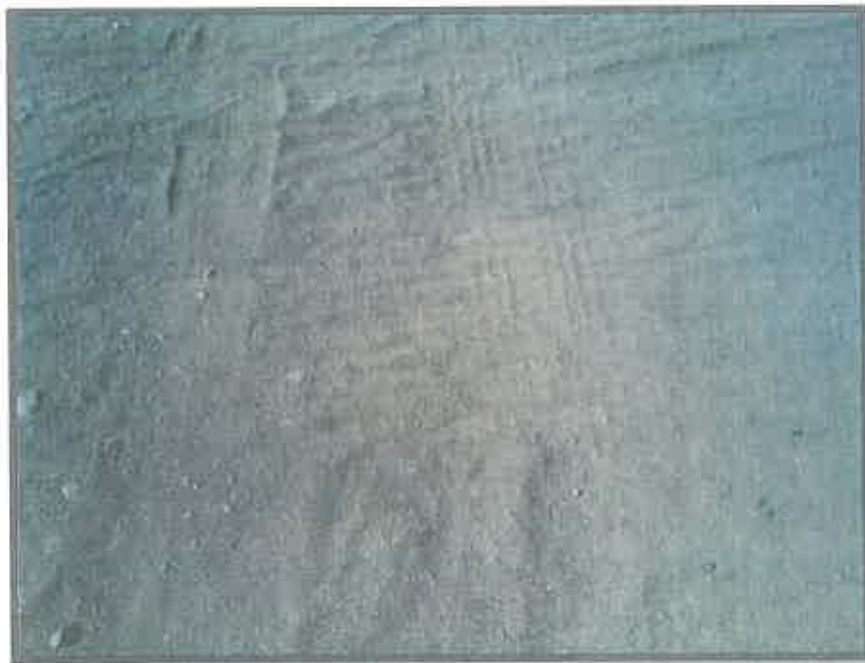
Figure 9: Coal dust along R555 road.
