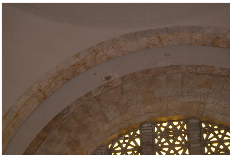
Figure 11. Dark patch above the entrance to the interior of the building (Photograph: M. Naudé 2020)
