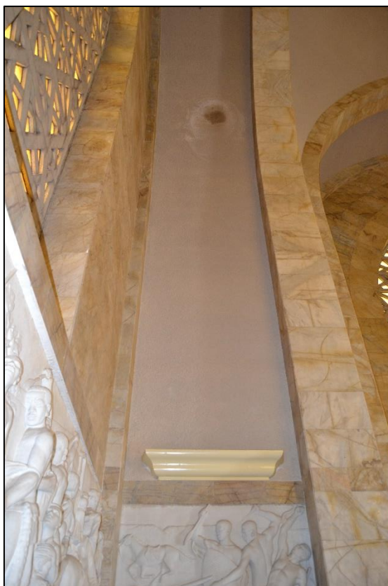
Figure 9. Colour patch on the curved ceiling along the south western corner (Photograph: M. Naudé 2020)
