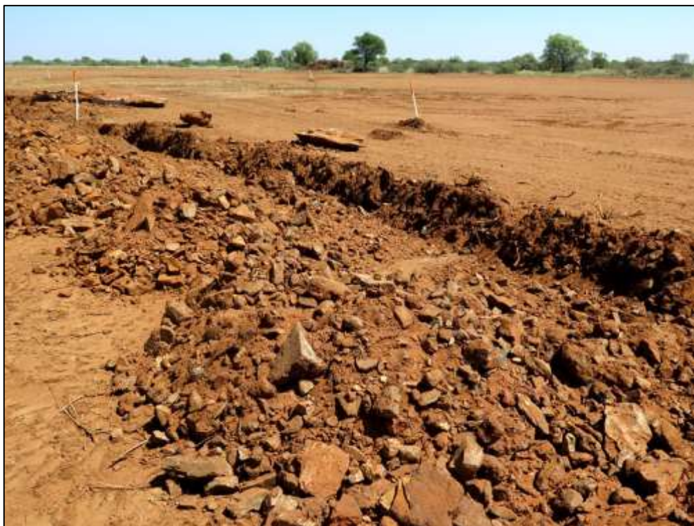
Figure 21: Coarse rubbly chert and carbonate material excavated from a trench just south of the HV Substation footprint (Loc. 345). The gravels here contain weathered as well as well-preserved small stromatolites such as those shown in the following four figures.
