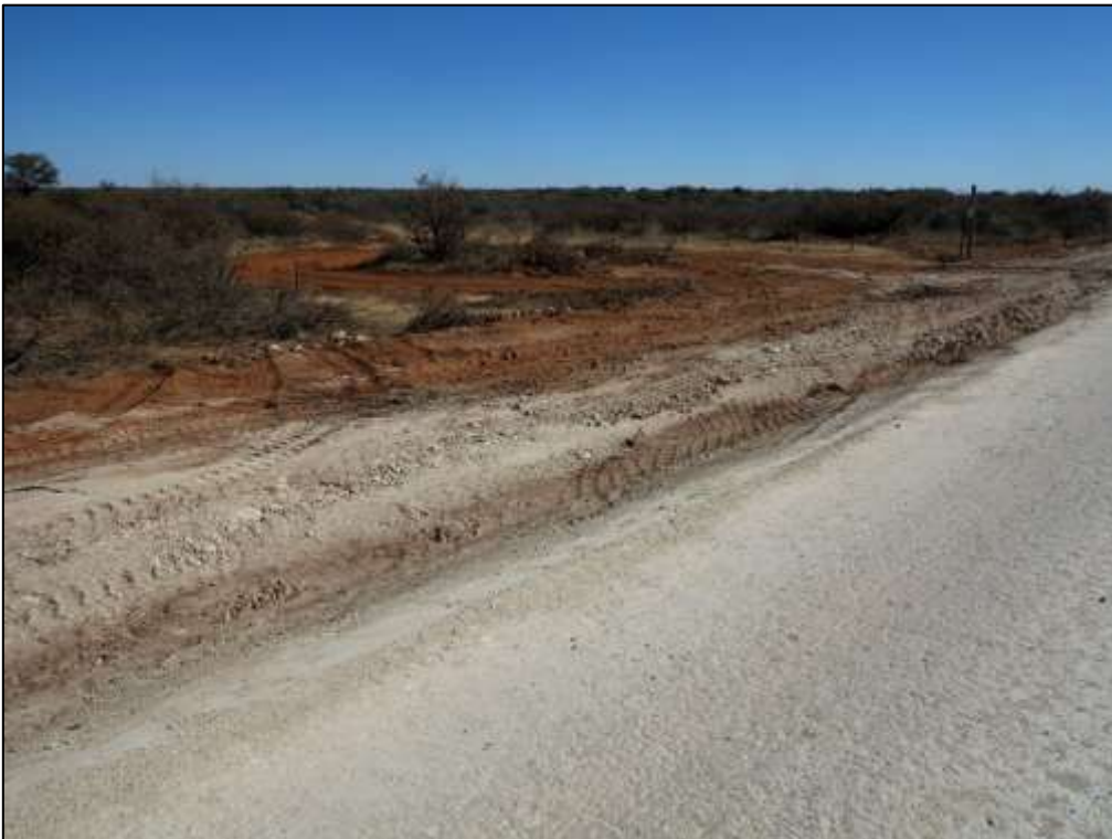
Figure 8: Surface disturbance by vehicle activity during the construction phase often extends well beyond the edge of the access roads. This is important to note for pre-construction heritage walkdown surveys for comparable developments.
