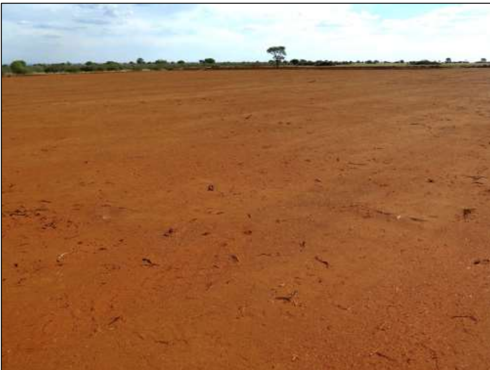
Figure 10: Following bush clearance, site levelling and spreading of gravelly soil, there is virtually no bedrock exposure left within laydown areas (here due SW of the Heritage Conservation Area).
