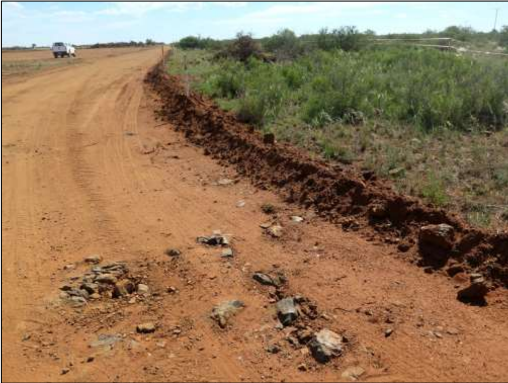
Figure 7: Surface scraping for the main access road that adjoins the HCA (background on RHS) has inevitably damaged silicified stromatolite domes (foreground).
