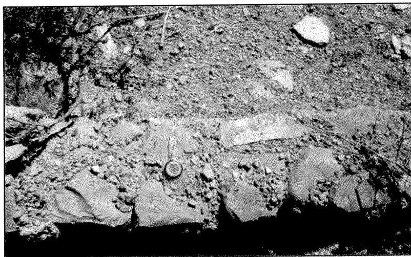
Fig. 10. Site CV 8. View from above with compass scale. The wall is approx. 35cm wide.
