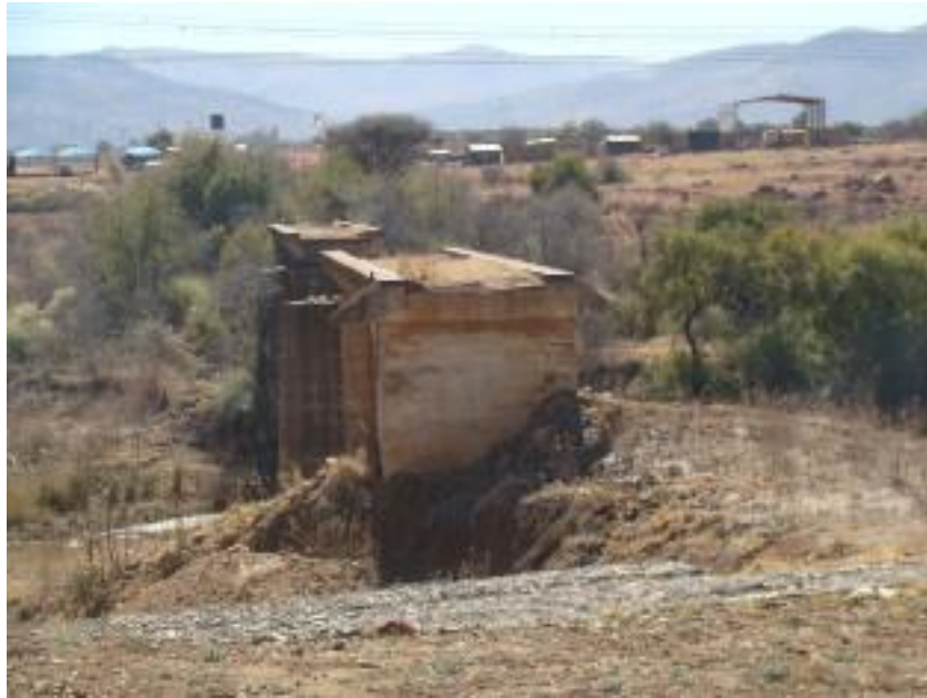
Figure 10: Old rail crossing NG04.
