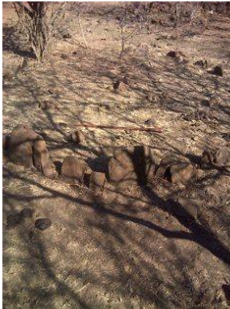
Figure 23: Hut foundations At NG25.
