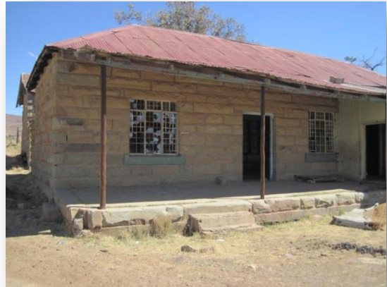
Figure 35 – View of the pitched corrugated iron roof of the old shop.
