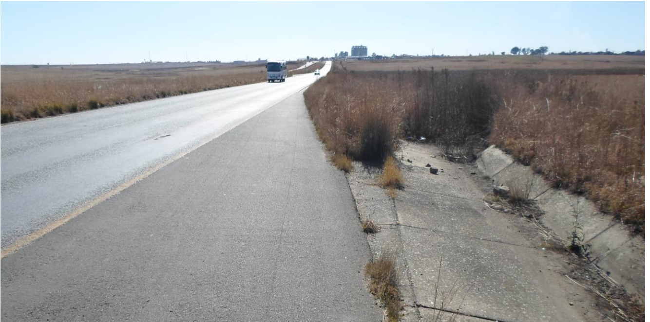
Plate 1: Photo 1: Showing proposed pipeline route along road servitude (Photograph © by Author 2022).
