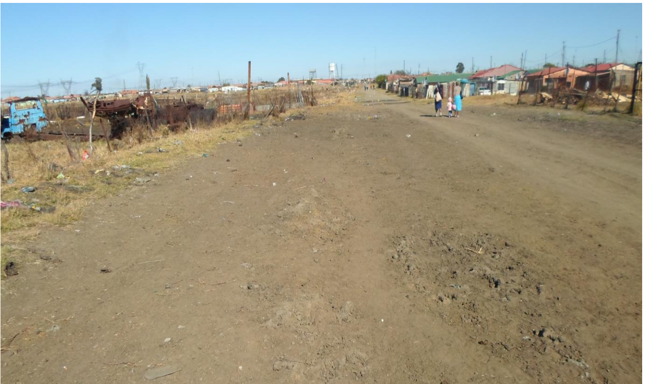
Plate 16: Photo 16: View of proposed pipeline route within a disturbed built-up area. (Photograph © by Author 2022).
