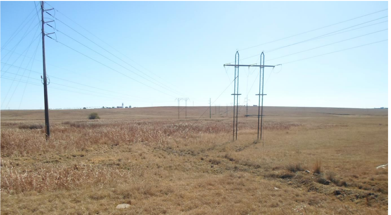
Plate 5: Photo 5: View of the proposed pipeline route along powerline servitude (Photograph © by Author 2022)
