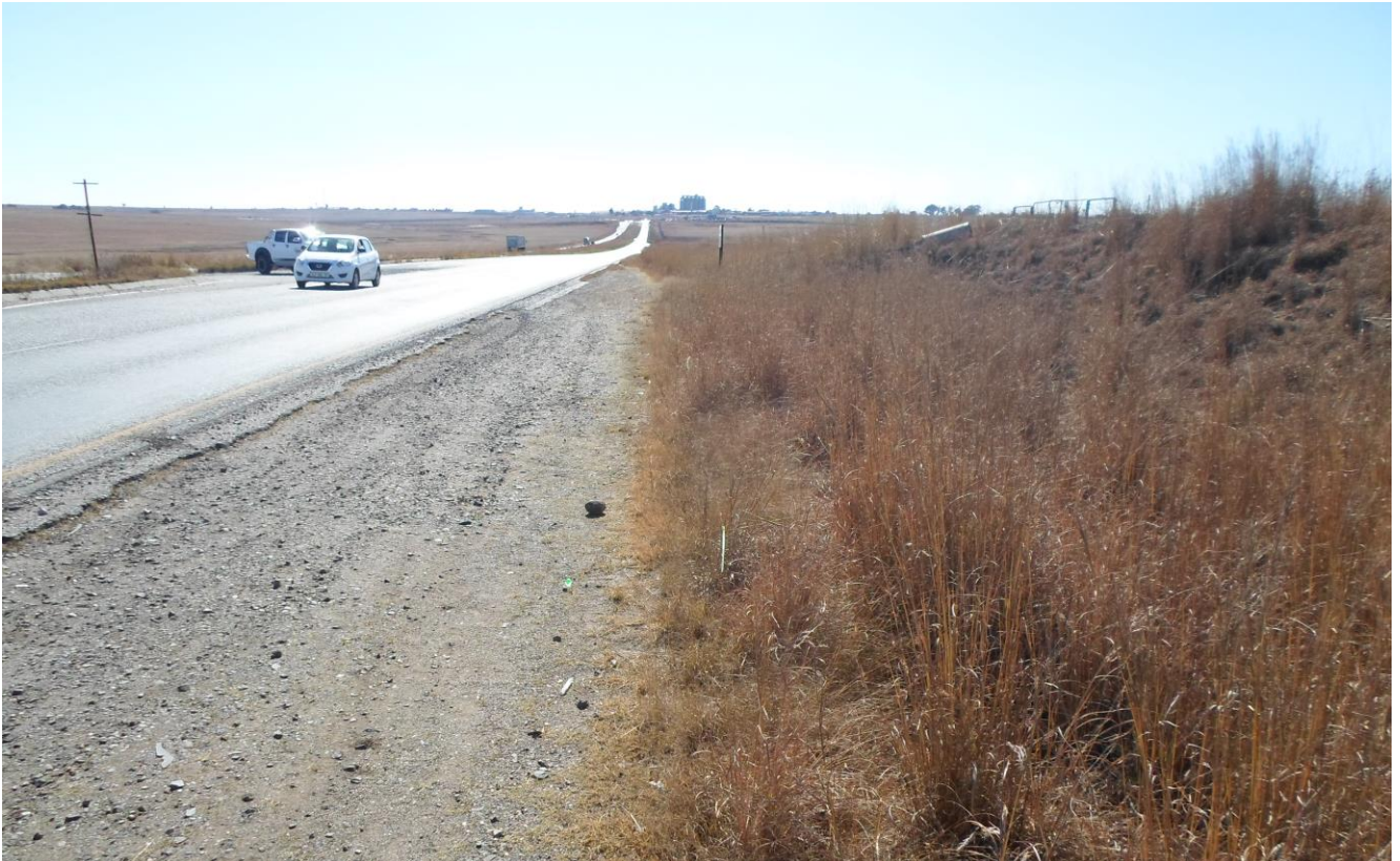
Plate 4: Photo 4: View of the proposed pipeline route along the road servitude (Photograph © by Author 2022).
