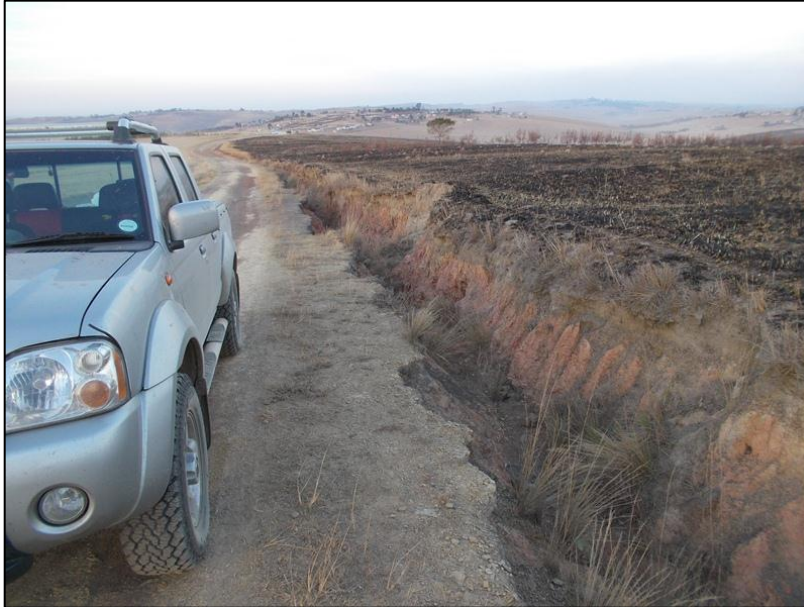
Photograph 1: Typical erosion feature near Dungu village.
