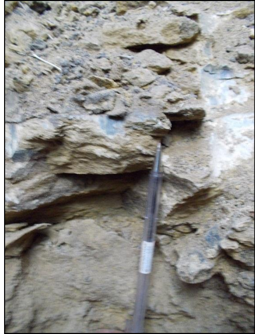
Note: Fractured and jointed structure of medium hard rock shale.
