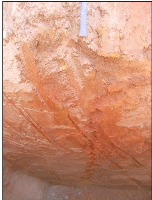
Note: Hole stopped TLB soft excavation.
