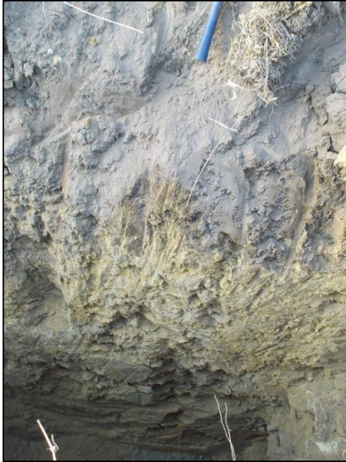
Note: Hole stopped TLB soft excavation.
