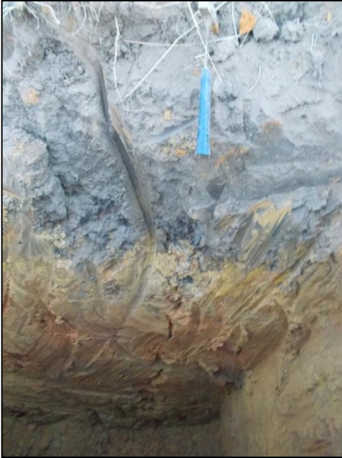
Note: Hole stopped TLB soft excavation.
