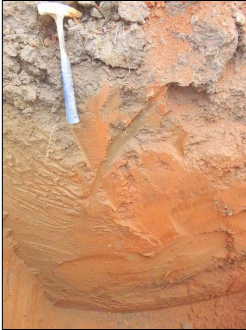
Note: Hole stopped TLB soft excavation.
