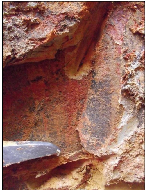
Note: Jointed structure in weathered shale.
