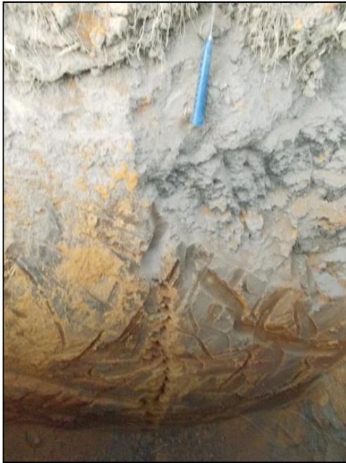
Note: Hole stopped TLB soft excavation.
