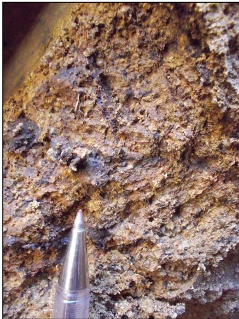
Note: Silty clayey residual dolerite in profile.
