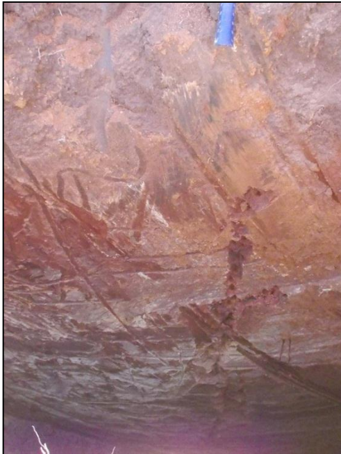
Note: Hole stopped TLB soft excavation.
