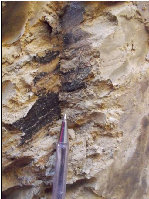
Note: Layered and jointed structure in highly weathered shale.
