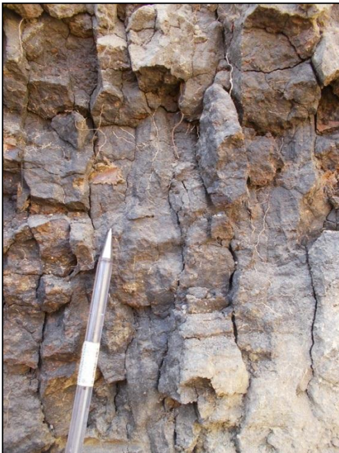
Note: Desiccation cracks in silty clay horizon.
