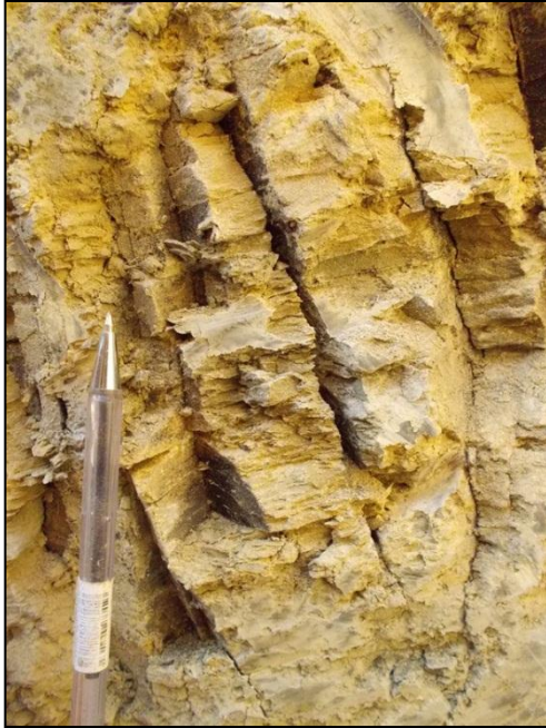
Note: Jointed and layered structure in highly weathered shale.
