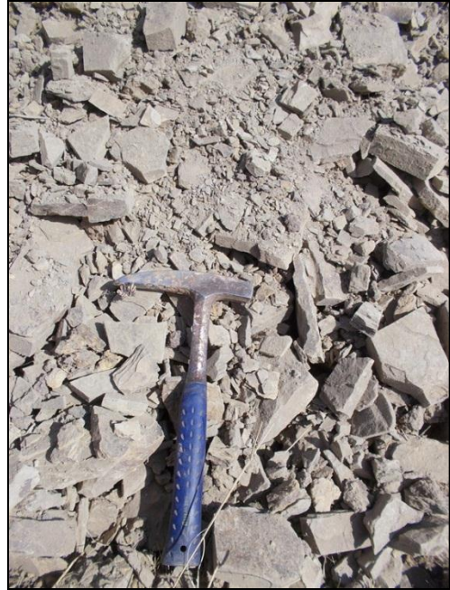
Note: Highly weathered shale fragments excavated.
