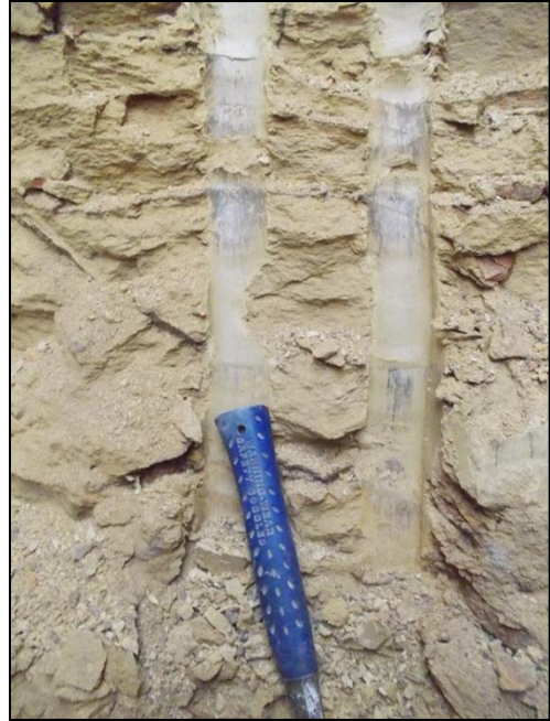
Note: Jointed and layered structure in soft rock shale at base.
