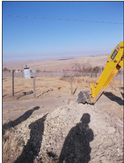
Note: View of down slope of village.
