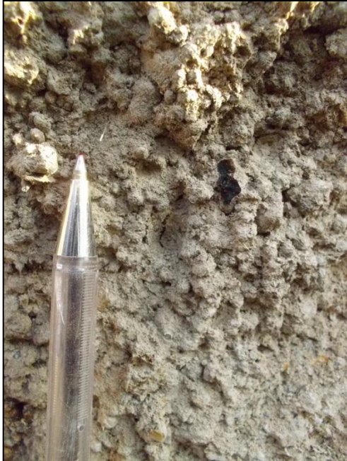
Note: Open structure in gravel of iron and manganese nodules.
