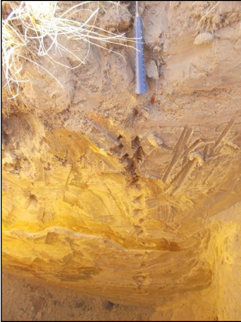
Note: Hole stopped TLB soft excavation.
