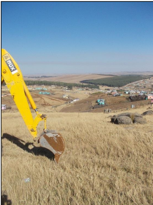
Note: View of site and slope on site.
