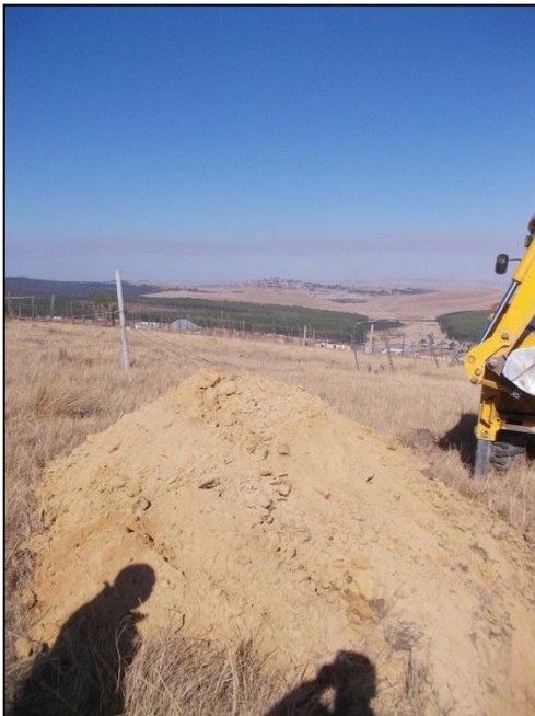
Note: Display of slope on site.
