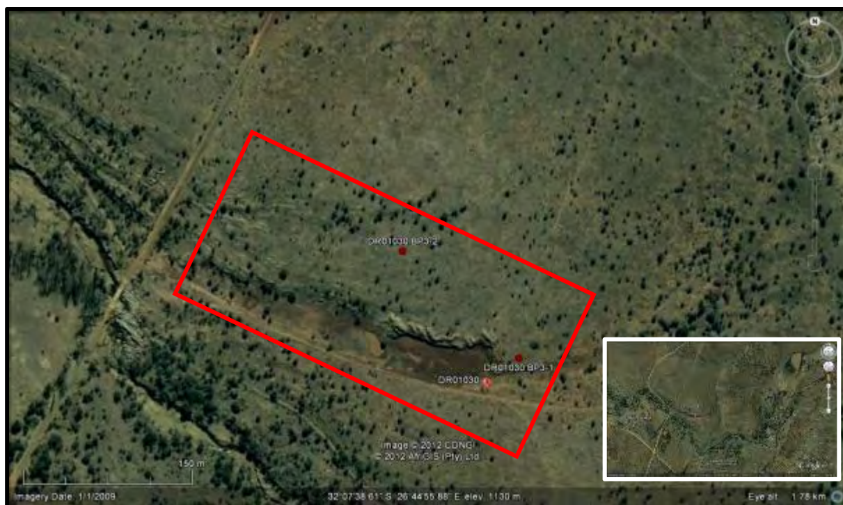
Figure 14. Map 8. Close-up aerial view of the borrow pit adjacent to the DR01030 near Poplar Grove.
