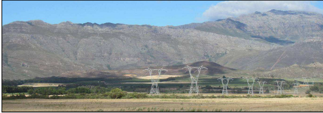
Plate 3: Existing transmission lines running more or less east west across the valley, cross the R45 in the area proposed for the wind farm.
