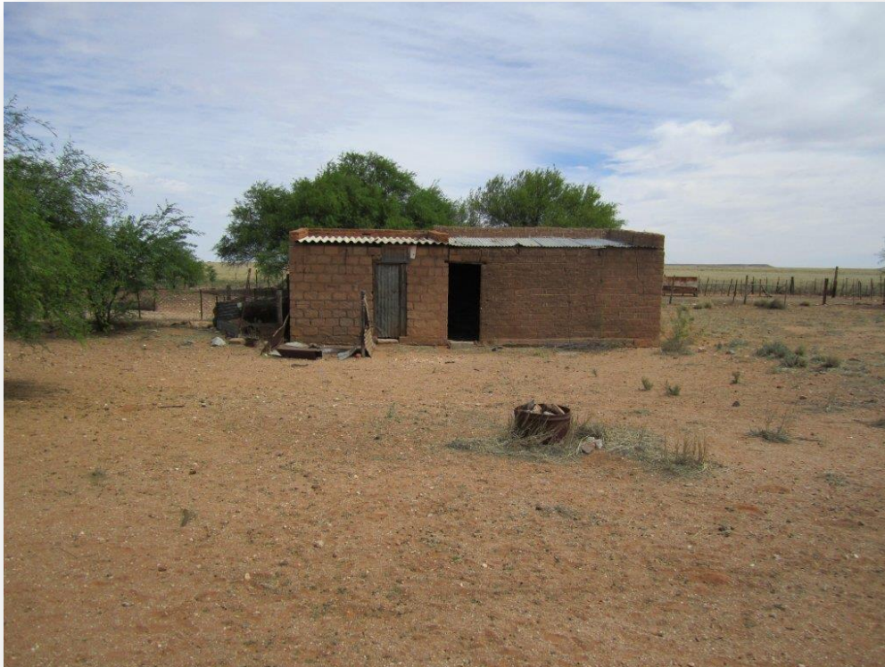
Figure 10 – Current structure on property
