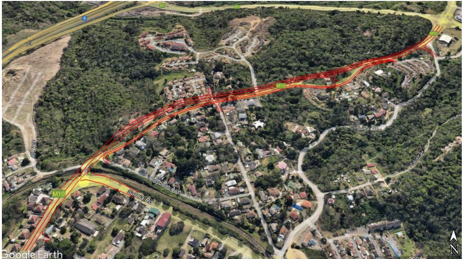
Figure 2: Closer view of section of road to be upgraded
