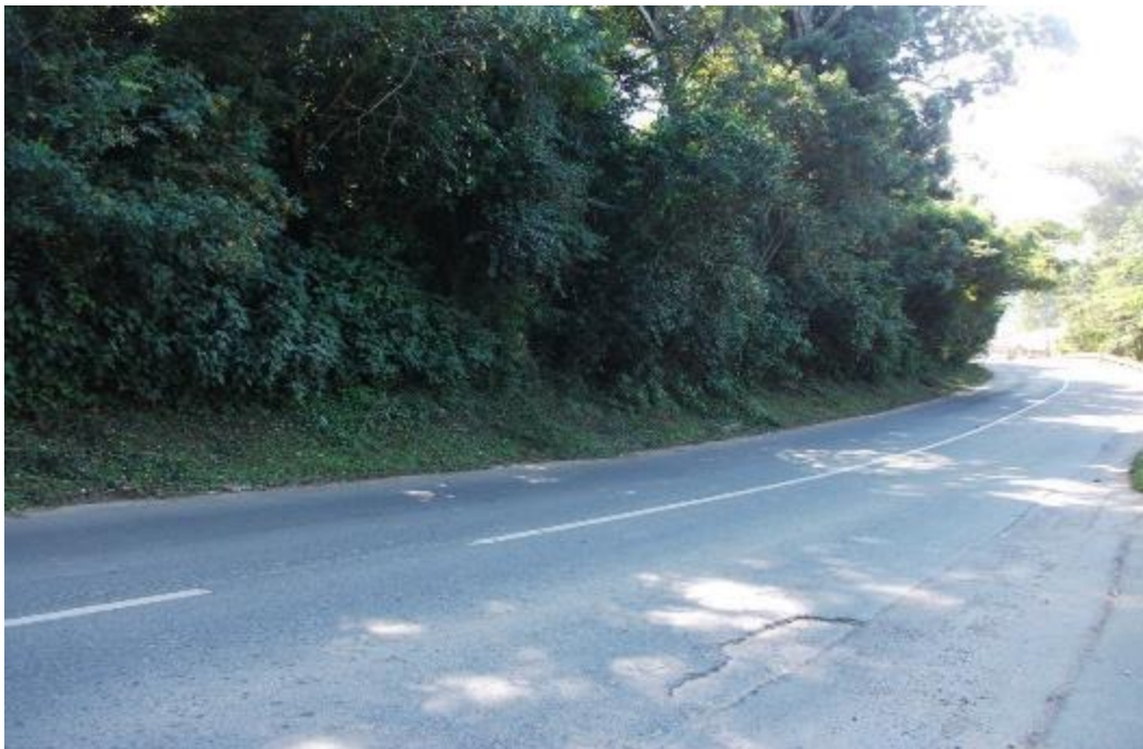
Figure 7: Vegetated section of Wakesleigh Road towards the M7 highway
