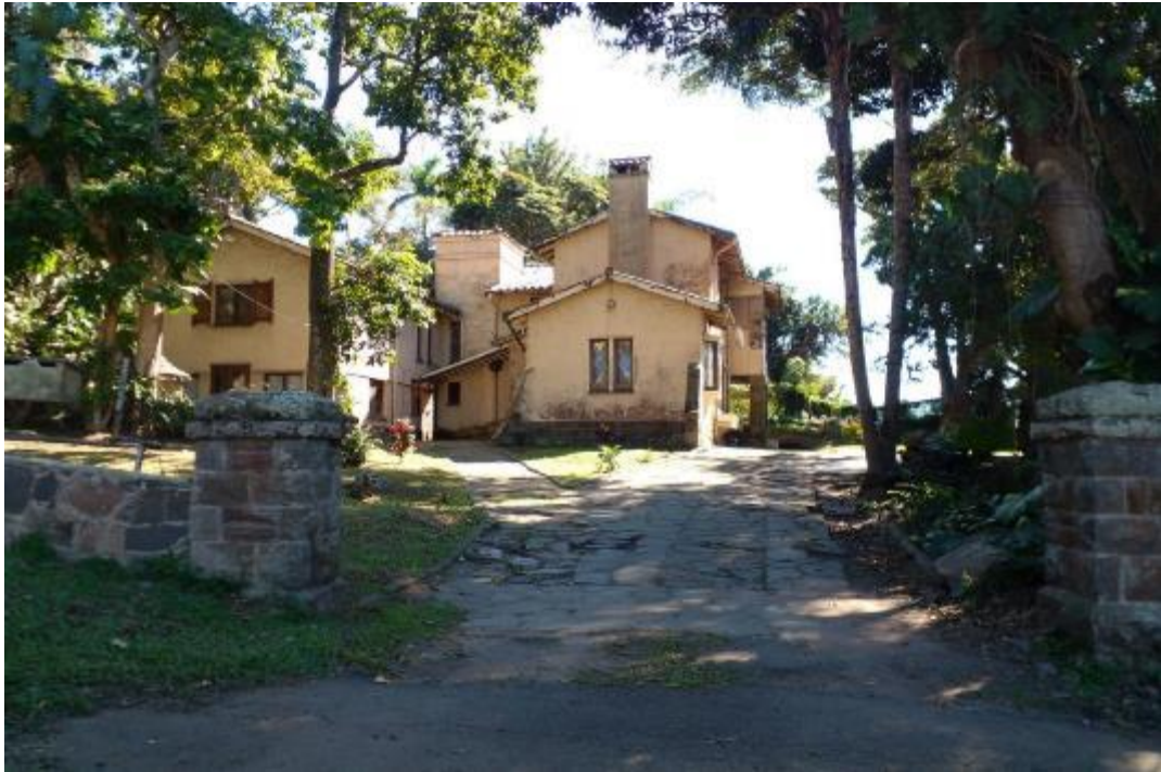
Figure 12: Dwelling and entrance gates that could be >60 years
