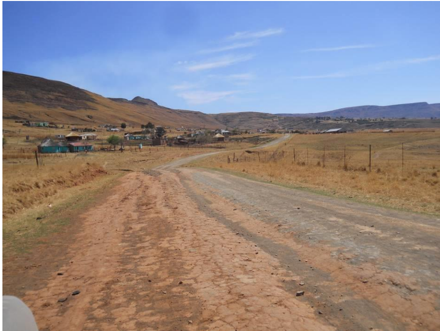
Figure 7.13 Most of the excavation for the pipeline will be into deep soils along the access roads (GPS 30 09 49.5S; 29 02 30.6E)
