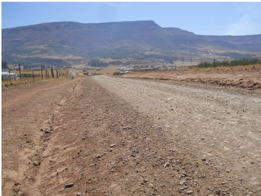
Figure 7.14 The southwestern section is also underlain by relatively deep soils where excavation for the pipelines will follow the access roads with very few outcrops of Burgersdorp Formation mudstone and no fossils were observed. (GPS 30 07 58.3S; 29 00 30.9E)
