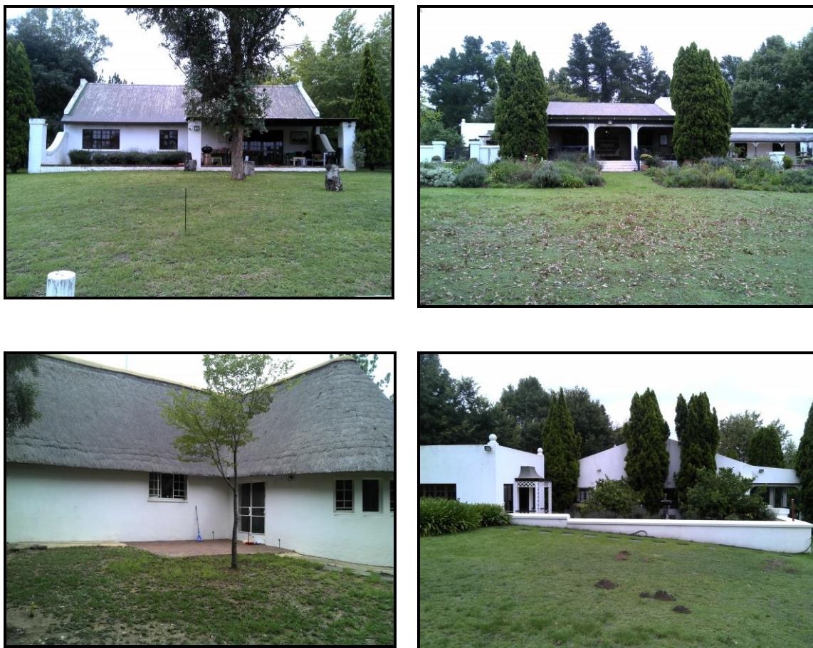
Figure 11: Structures in the study area.
