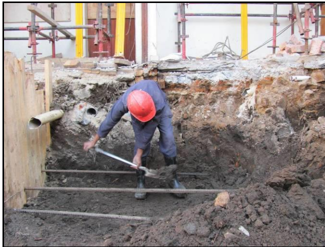
Plate 10: Steel rods were hammered into the deposit to prevent soil collapse.
