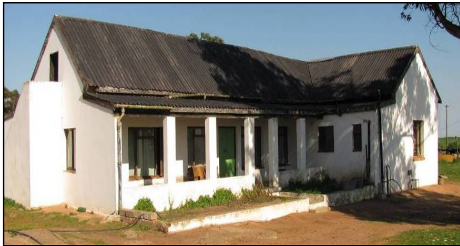
Plate 13: Front view of the Klipheuvel farmhouse showing the addition to the front, the modern windows and pillars.
