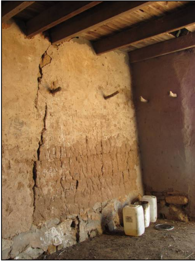
Plate 15: Inside of barn showing wooden ceiling, mud brick walls and wooden pegs.
