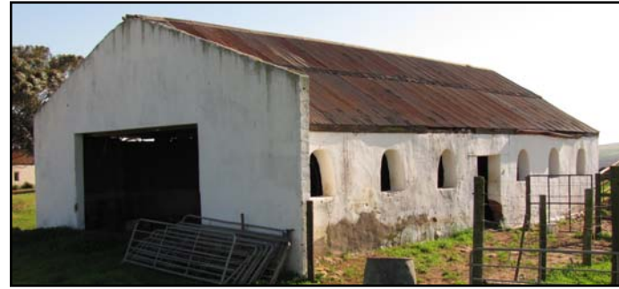
Plate 16: 20 th century barn with arched windows
