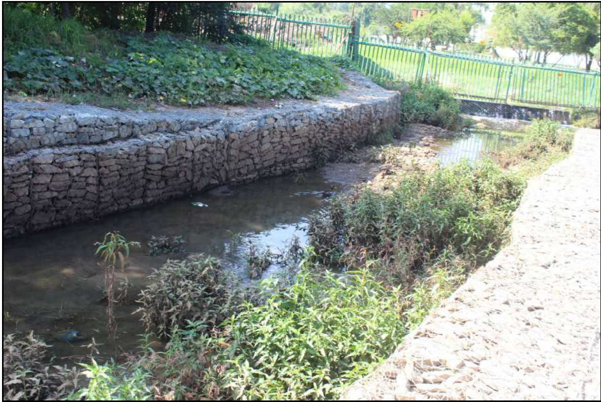
Figure 7: View of the previously rehabilitated river bank on the Derren wood stream
