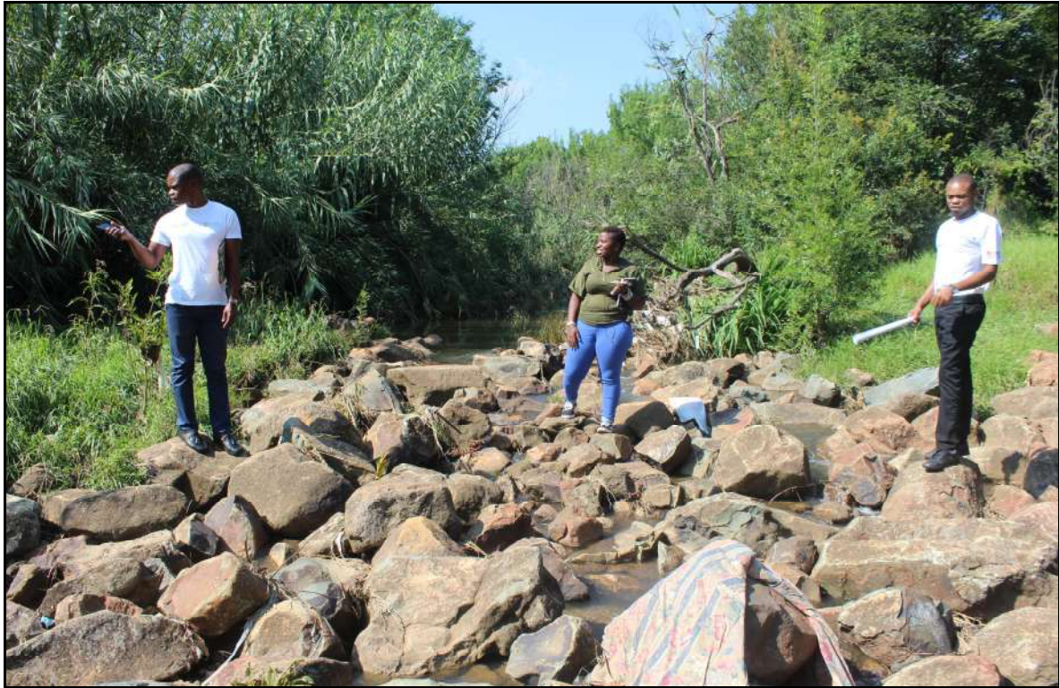
Figure 5: Flood control measure, where rocks weir have been used to reduce the velocity of floodwater
