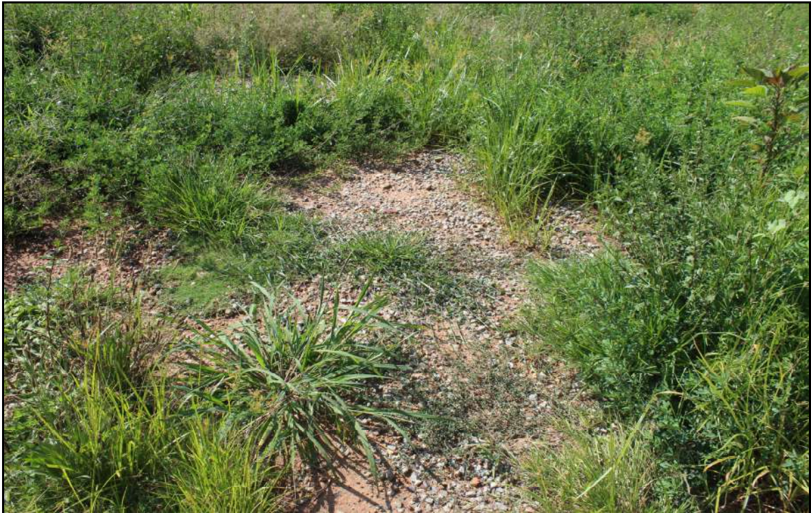
Figure 9: Surface disturbances (crushed stones)
