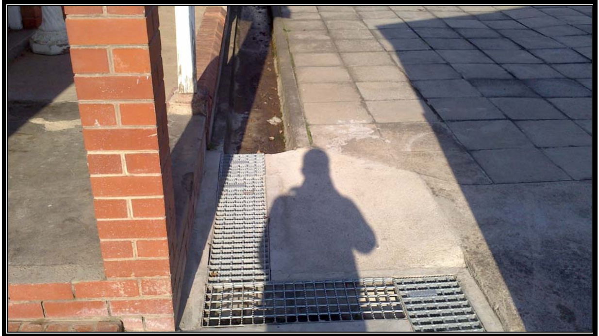
Photograph 11: View of steel grating over portion of storm-water channel
