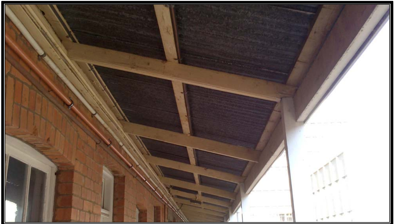
Photograph 8: View of roof to verandah
