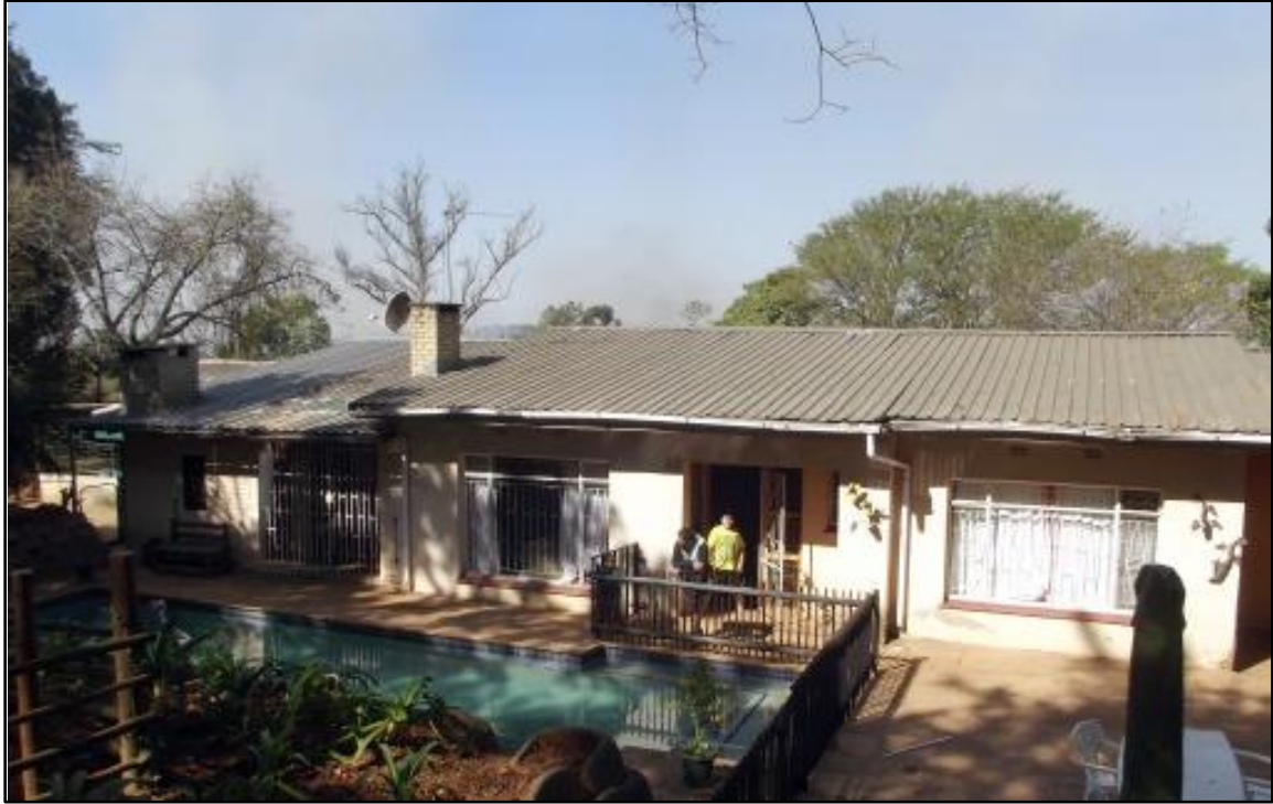
Fig. 5. Site WAH 2. The section to the West of the original structure was added later on.
