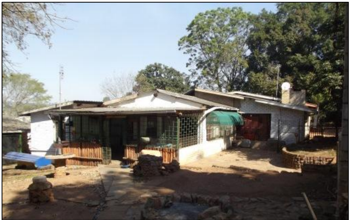
Fig. 4. Site WAH 2. The Stander house from the East. In front is the older structure and addition to the rear (West).
