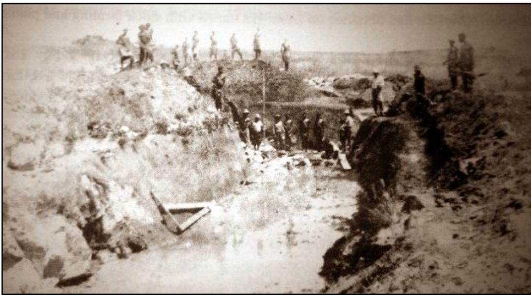
Fig. 4.2. Early settlers constructing an 25km water canal from the White River to irrigate their farms (taken from Bornman, 2015).
