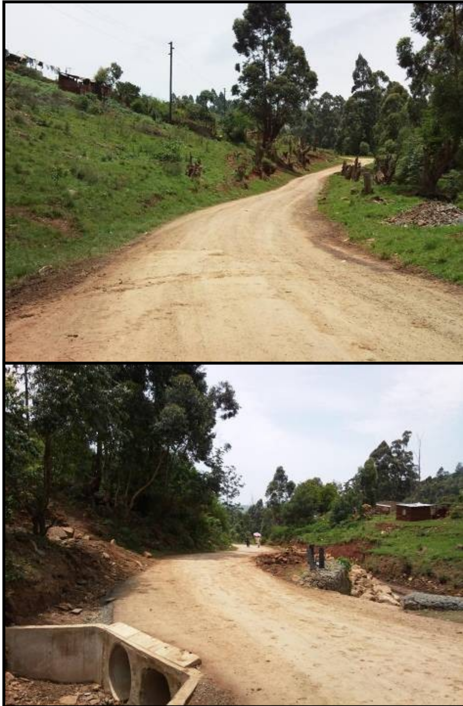
FIG. 4: CURRENT CONDITION OF THE PROPOSED ROAD UPGRADE
