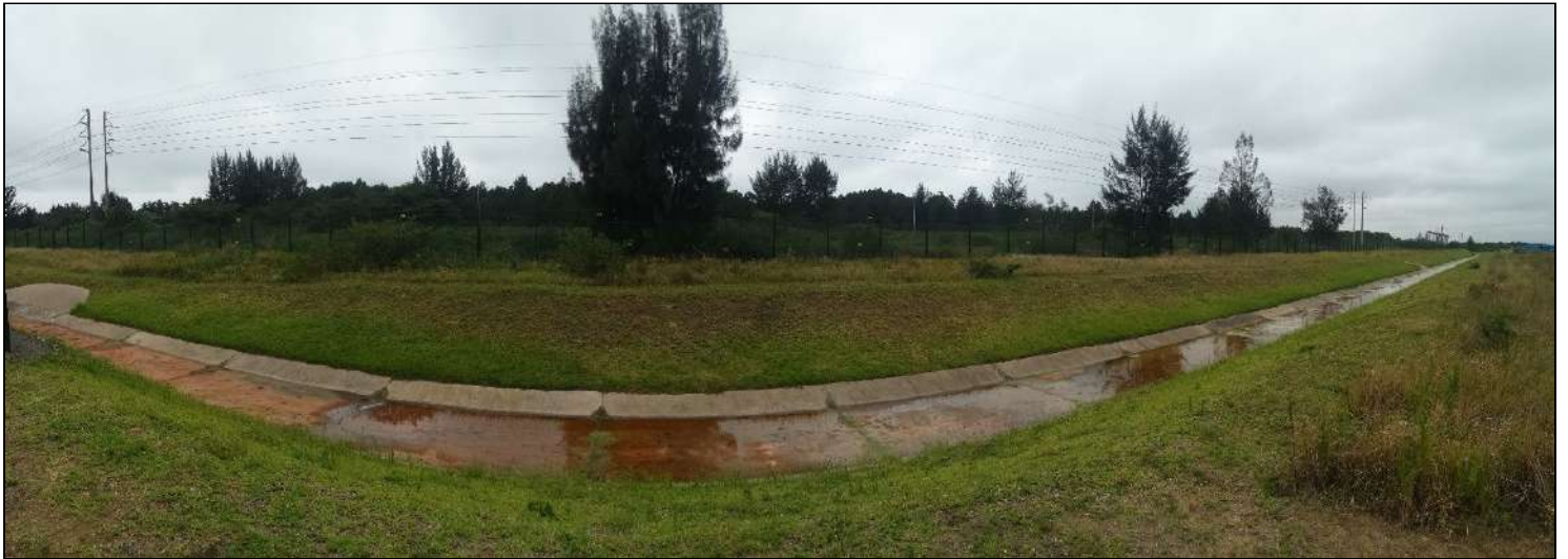
Figure 7.3 V drain channels to drain previous swampland.
