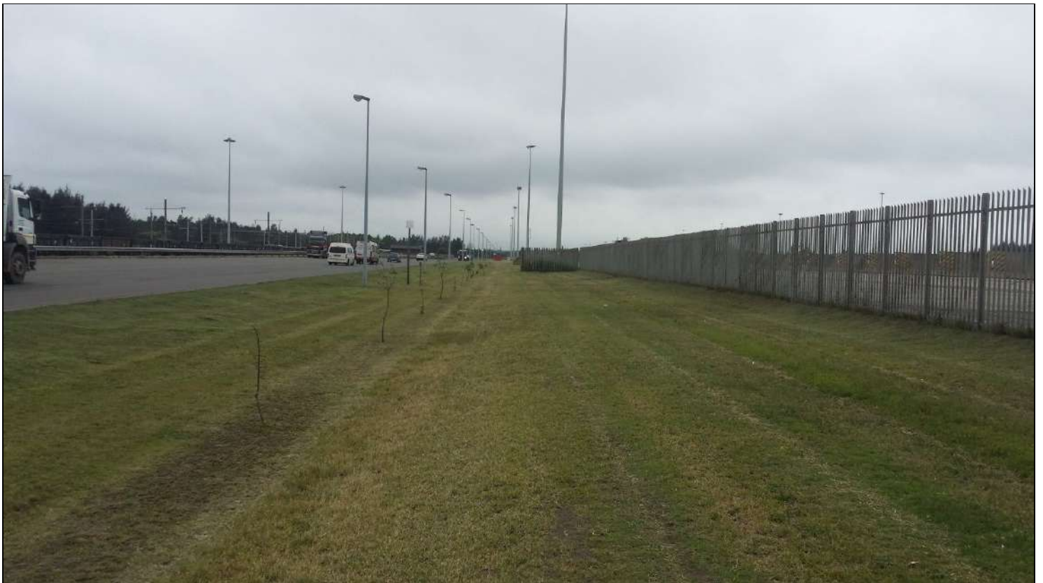
Figure 7.10 Existing infrastructure along pipeline route
