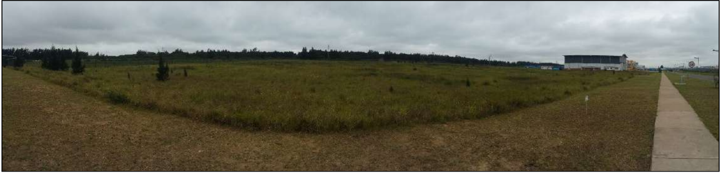
Figure 7.2 Infrastructure layout on grasslands. Note emerging pioneer Casuarina trees on disturbed basement.
