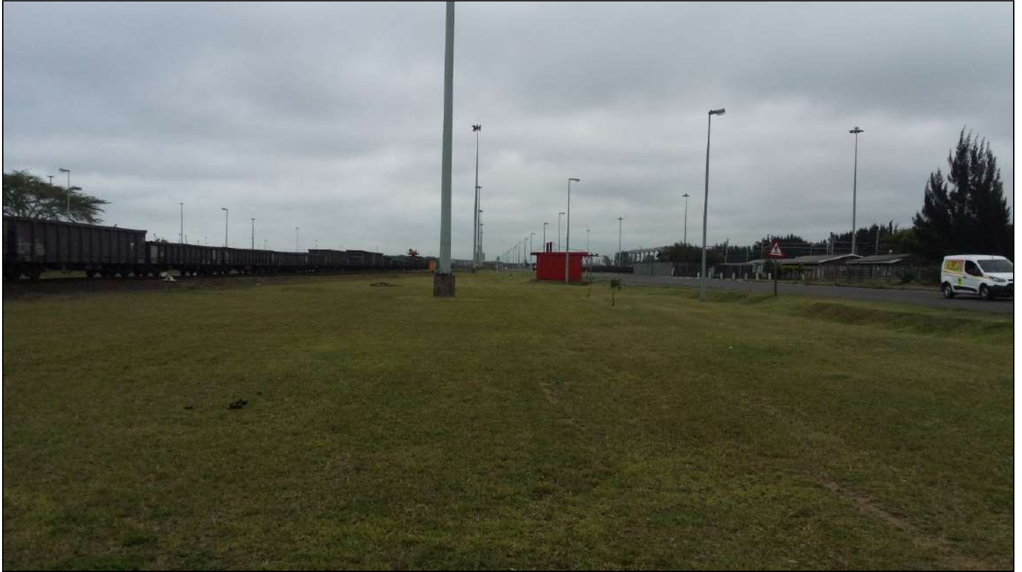
Figure 7.9 Existing infrastructure along pipeline route
