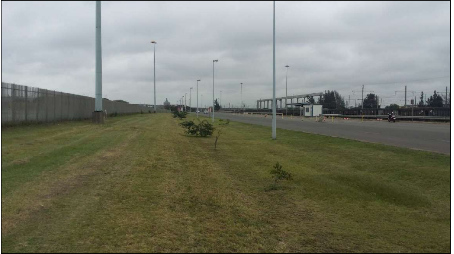
Figure 7.11 Existing infrastructure along pipeline route
