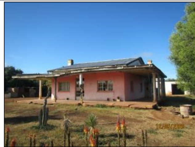
Figure 28 - View of the northern façade.
