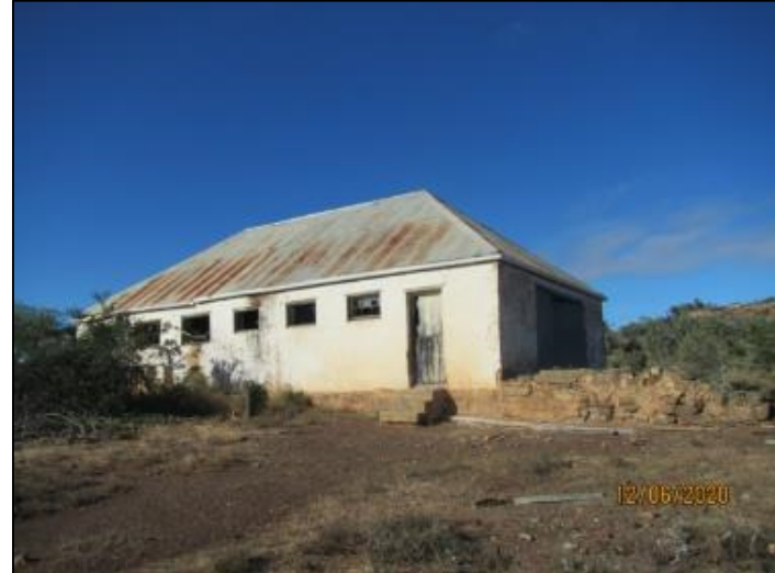
Figure 25 - View of the northern façade.
