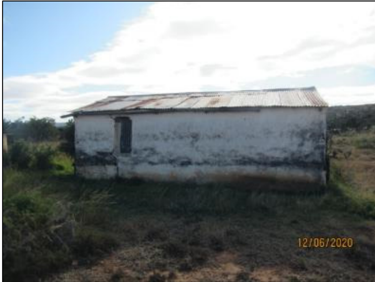
Figure 60 - View of the southern façade.
