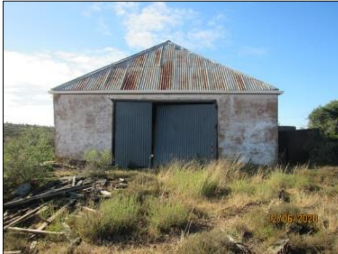
Figure 24 - View of the western façade.
