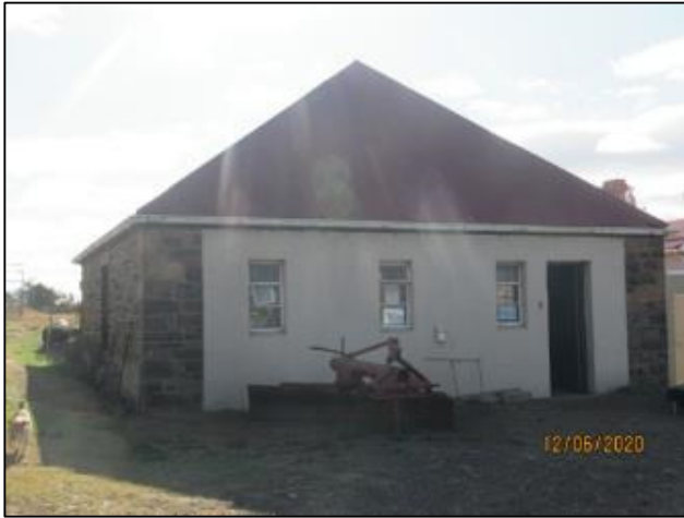
Figure 37 - View of the garage located next to the main farmhouse.
