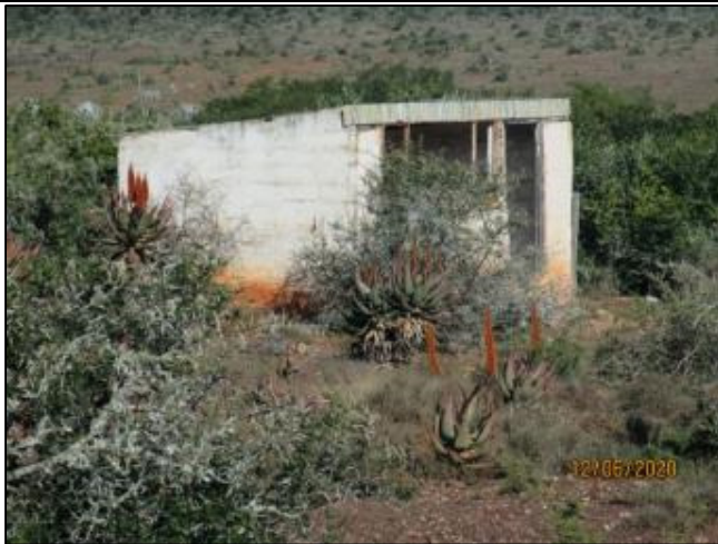
Figure 29 - View of the outbuilding.
