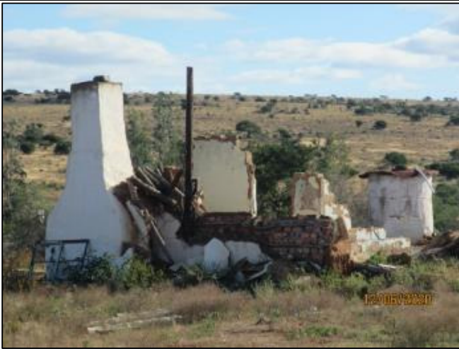
Figure 49 - Demolished labourer house.
