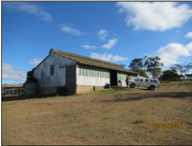
Figure 41 - View of the bigger shed.
