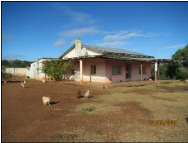
Figure 27 - View of the north-eastern corner of the house.
