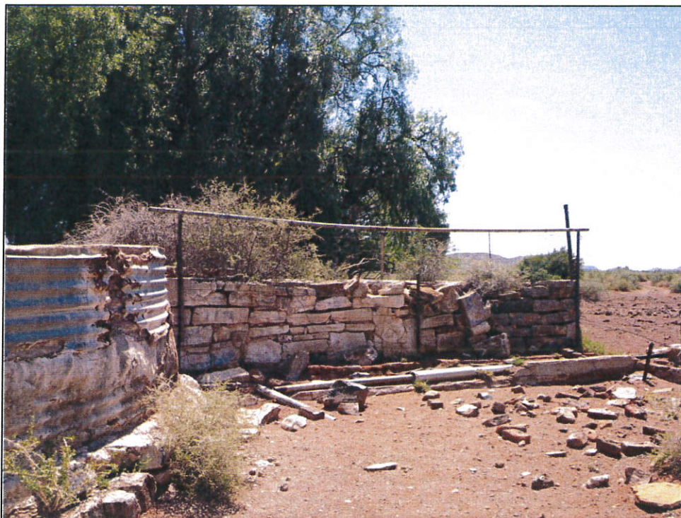
Figure 43. Livestock Enclosure and Dam
