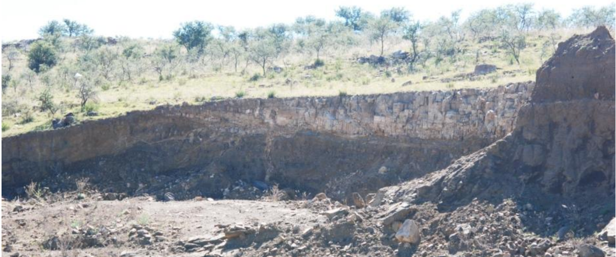
Figure 4. Metamorphosed Katberg Formation sandstones overlying a dolerite sill, exposed at the back of borrow pit 5.
