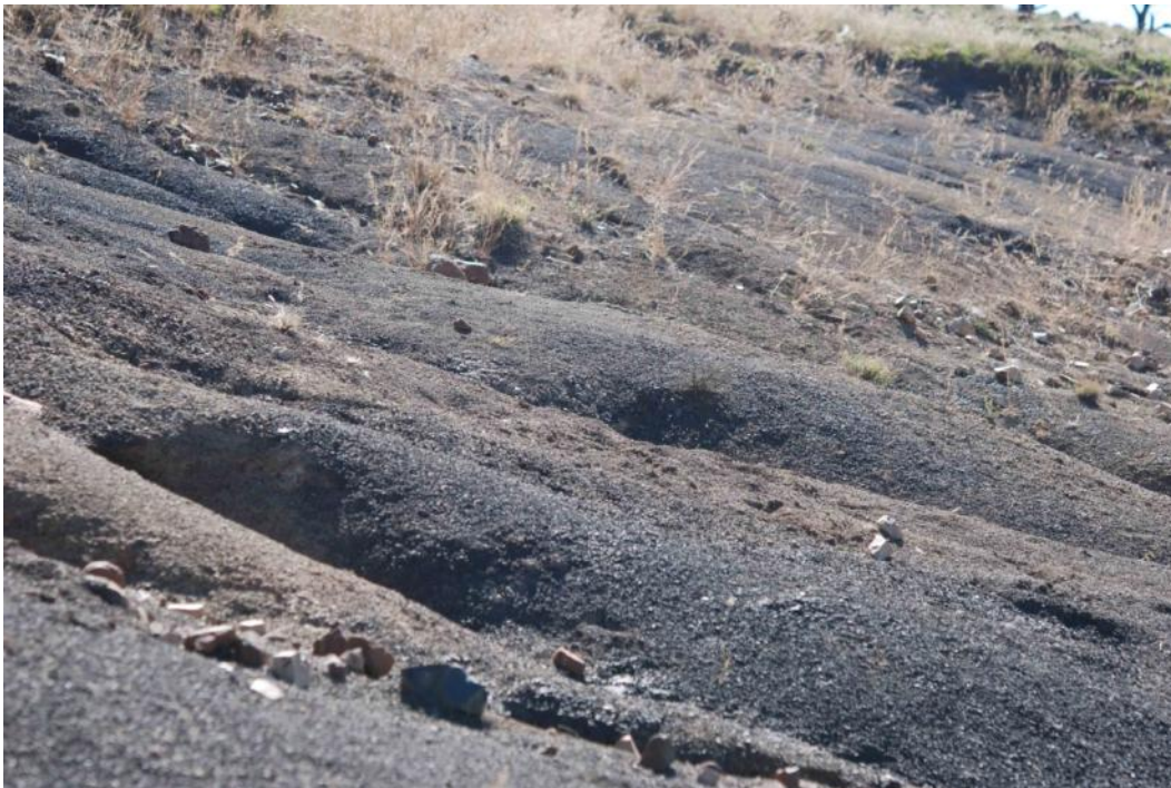
Figure 11: Burgersdorp Formation mudstone altered to bluish colour by metamorphism at borrow pit 3.
