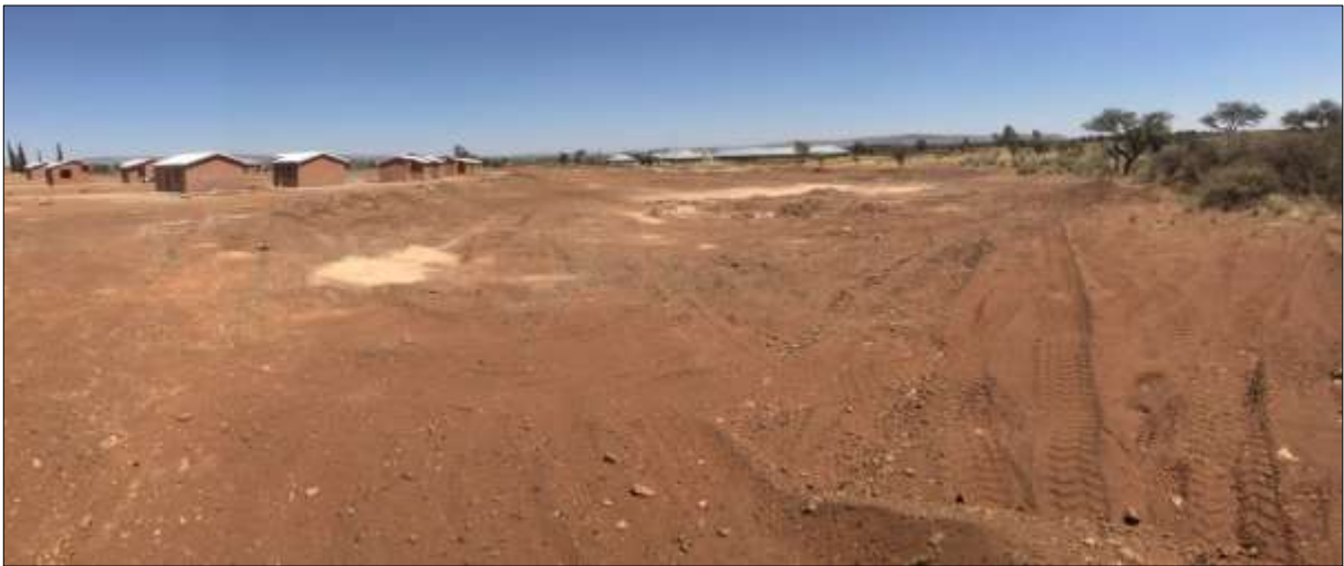
Figure 12. View of the development site facing west, with the Wrenchville School in the background
