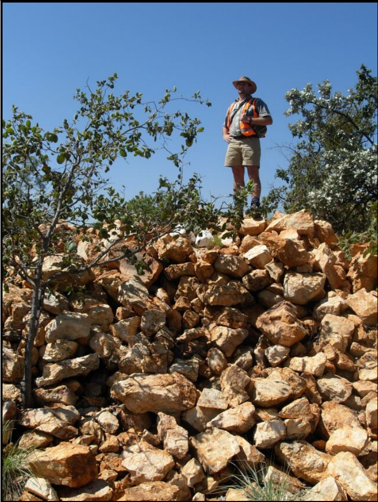
Figure 3: Photo of blockhouse foundation
