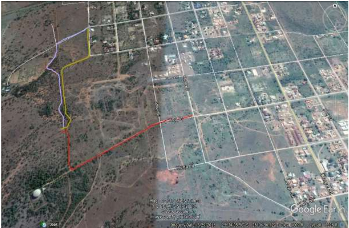
Fig.2: Close view of Alternative Access Roads (Google Earth 2016 – Image date 29/05/2016).
