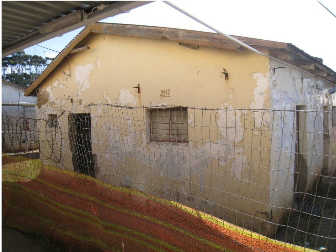
Fig 47: The Old Physiotherapy Block from the Kitchen building above it
