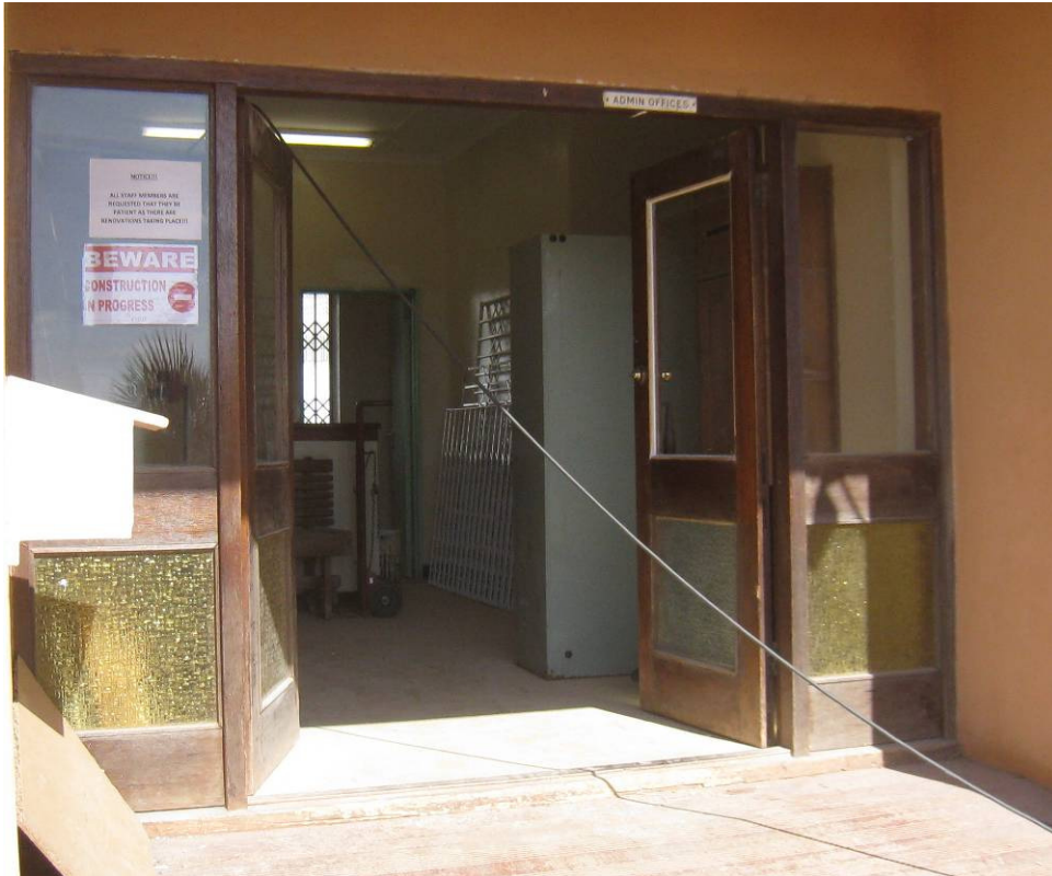
Fig 17: Front entrance doors to the Administration Block
