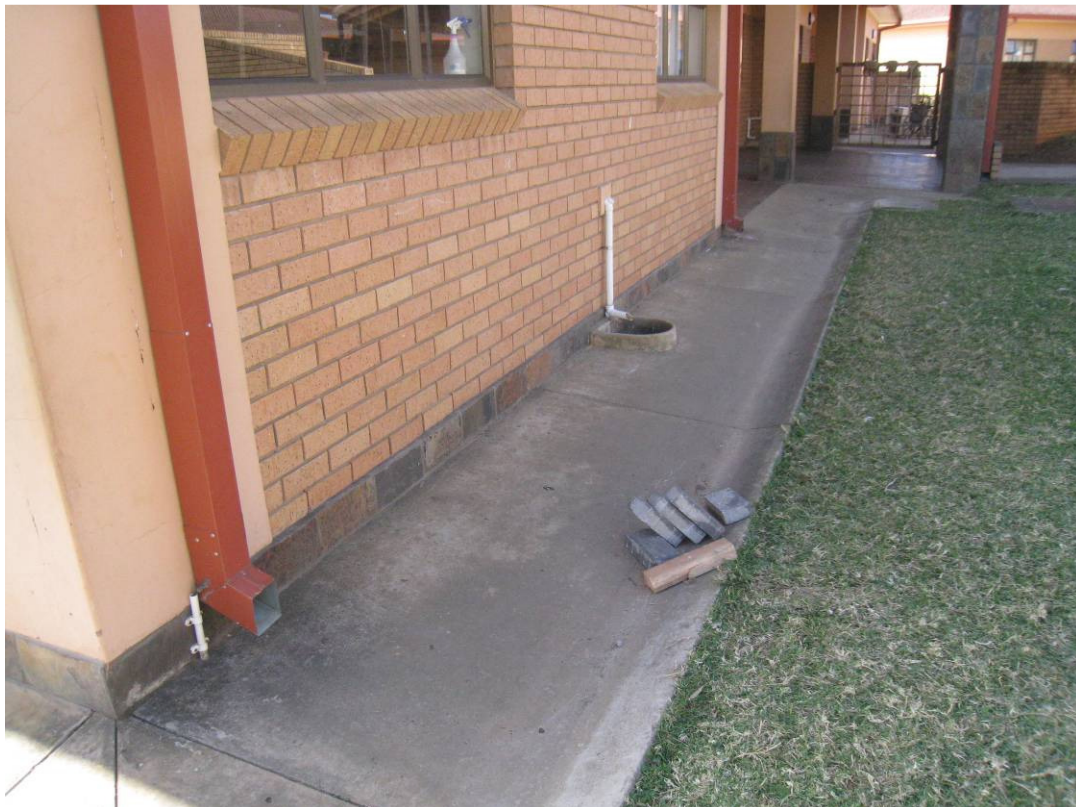
Fig 35: Detail showing material construction and condition of Paediatric Department
