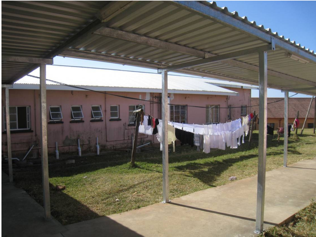
Fig 37: Staff Accommodation, lower level
