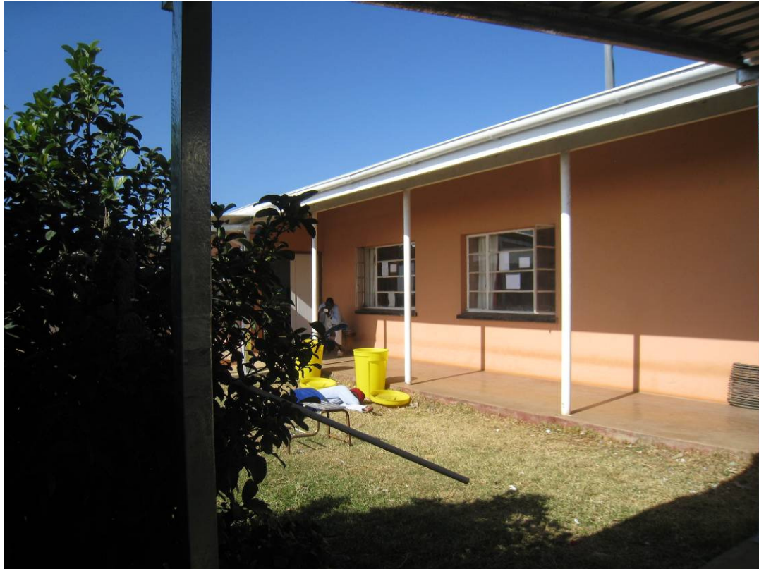
Fig 21: Front veranda, recently refurbished
