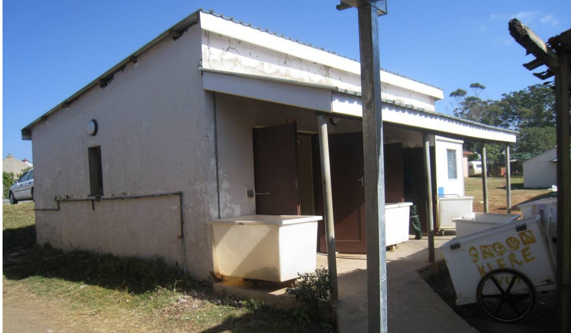
Fig 27: The Laundry Block from the north east
