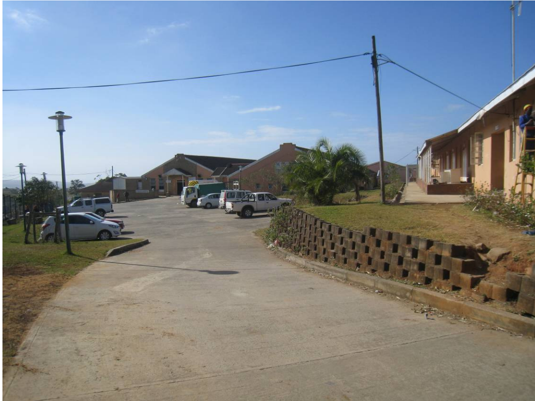
Fig 9: View along the entrance terrace with the Administration Block to the right, the Physiotherapy Block to the centre and the Outpatients Department to the left
