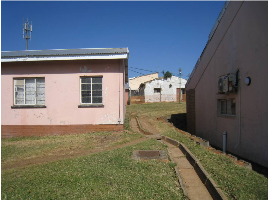
Fig 49: View up between the Physiotherapy block on the right and Nurses accommodation on the left to the old Matron's building in the background.
