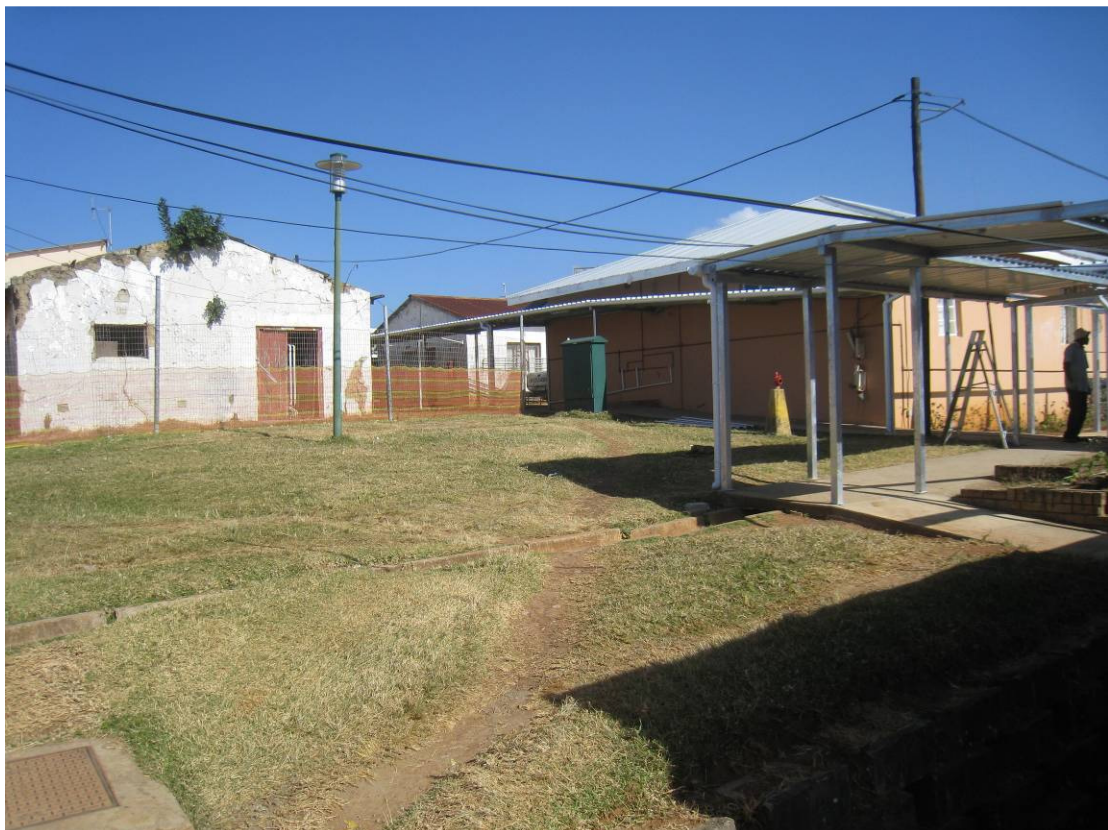
Fig 50: Old Physiotherapy Block from the north east with the Old Stores directly behind it and the end of the Administration Building to the right
