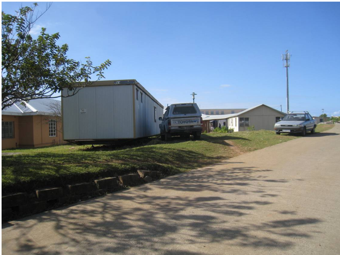
Fig 10: General view in the same direction at the rear of the Administration Block which is on the left and a prefabricated building in the distance
