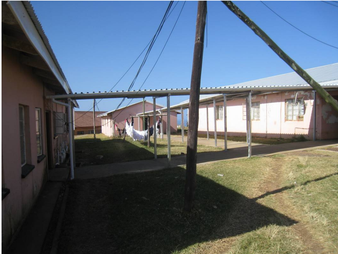
Fig 39: Staff Accommodation (all three buildings) showing connecting walkways
