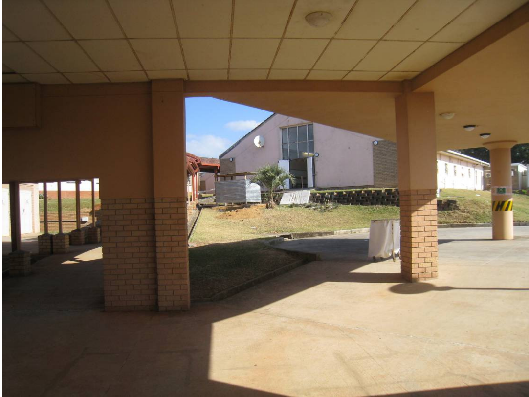
Fig 31: Rear of the Outpatients Department from the entrance to the Paediatric Block
