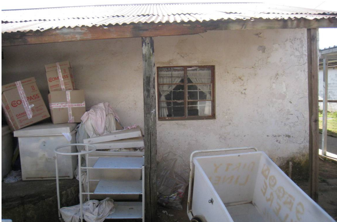
Fig 25: The Old Stores from the Laundry Block
