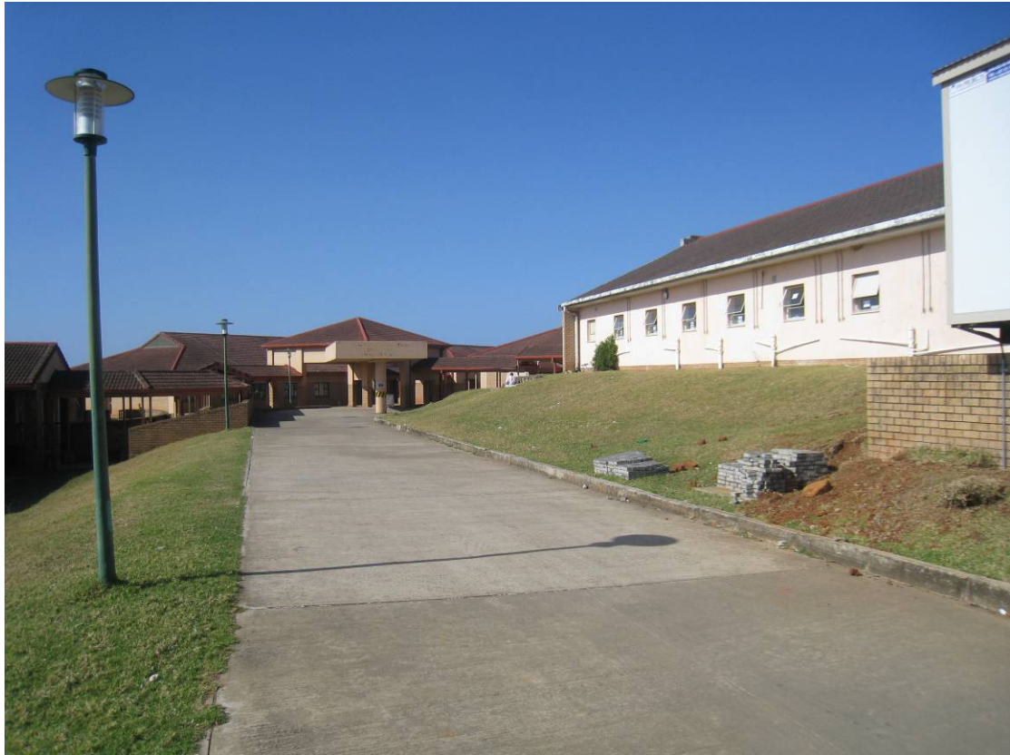
Fig 11: View along the contour to the passages connecting the Paediatric Wards (left) the General Wards (ahead) and the Outpatients Department (right)
