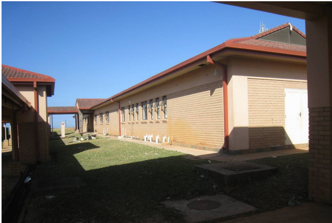
Fig 44: View of General wards
