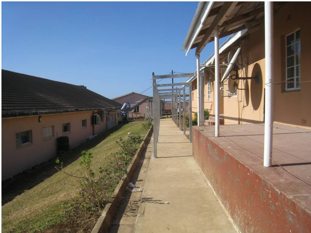
Fig 22: View along front veranda with Physiotherapy Block to the left and Nurses Accommodation in the background
