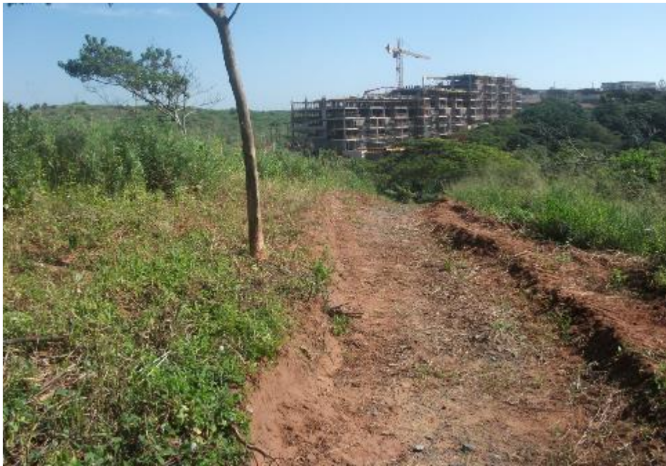
Figure 8: Looking over project site towards development on northern boundary of site
