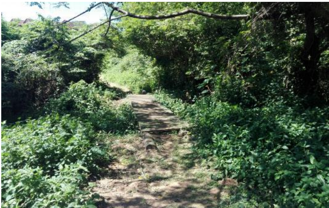
Figure 15: Wooden bridge over drainage line
