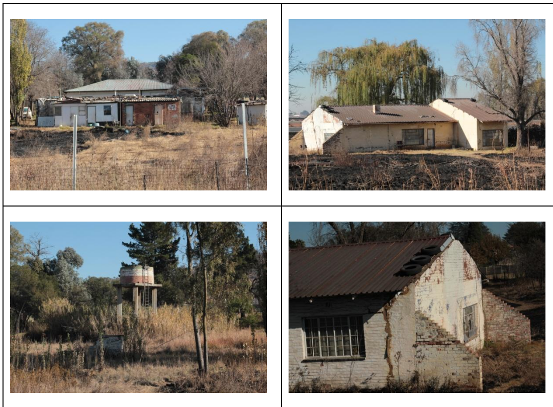
Fig. 8. The various structures on the western portion of the study area.
