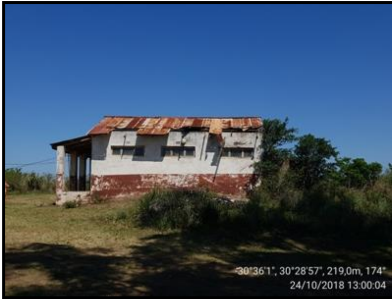
FIG. 19: GENERAL VIEWS OF THE VUKUZHAKELE GENERAL STORE
