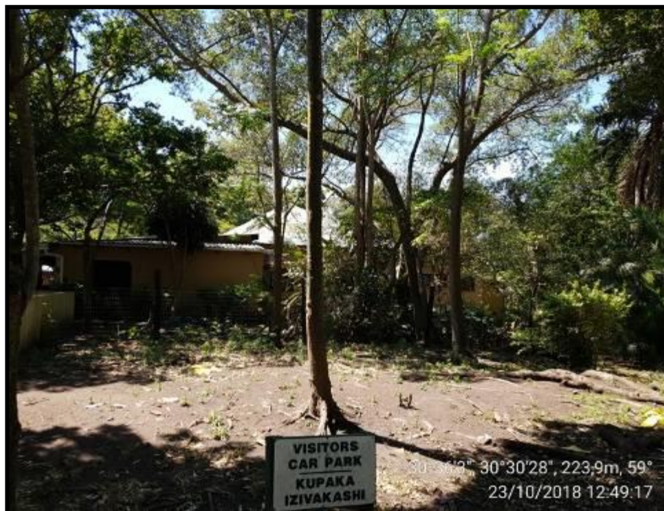
FIG. 13: THE NEUK BUILDING
