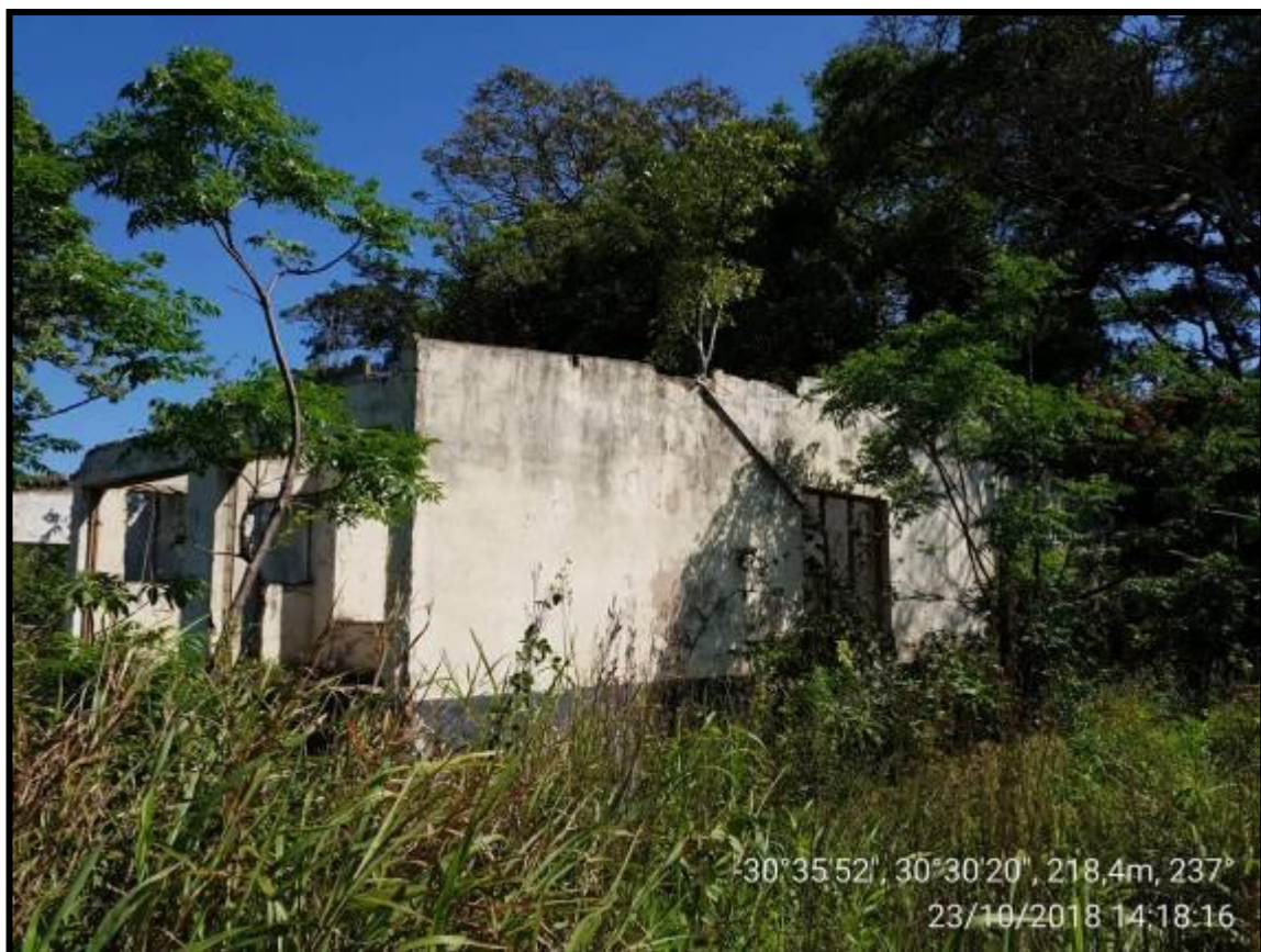
FIG. 14: BUILDING AT MUCKLEBRAES
