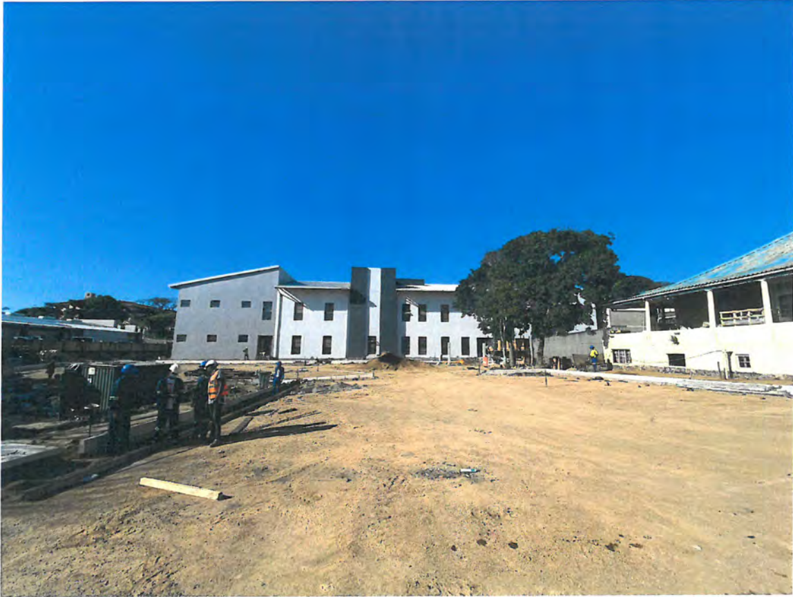
View of leveled parking from northern side
