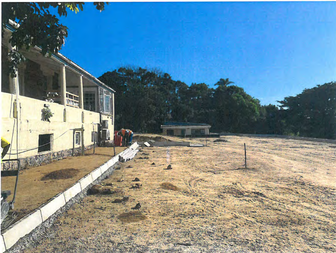
View of levelled parking form southern side
