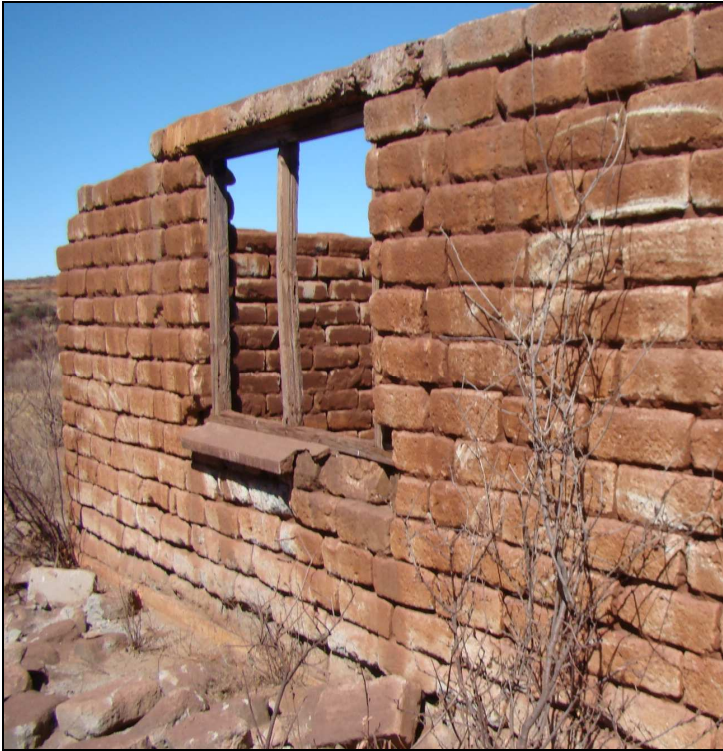
Fig.11 Wooden windowframes in the concrete walls.
