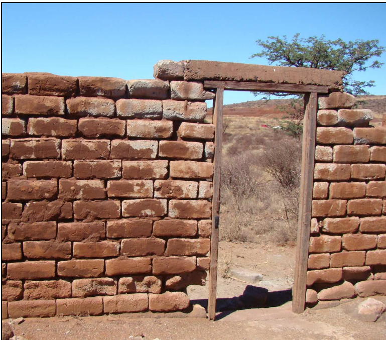
Fig.10 Wall with concrete lintel and wooden door frame.
