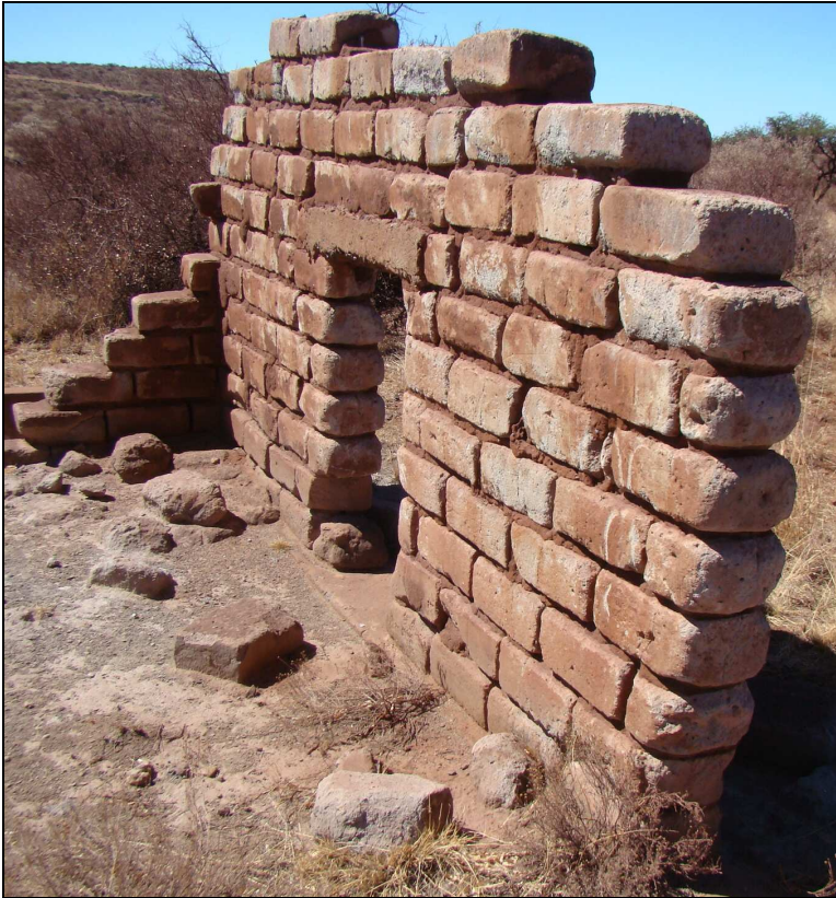
Fig.9 Wall with low concrete lintel at Demaneng.
