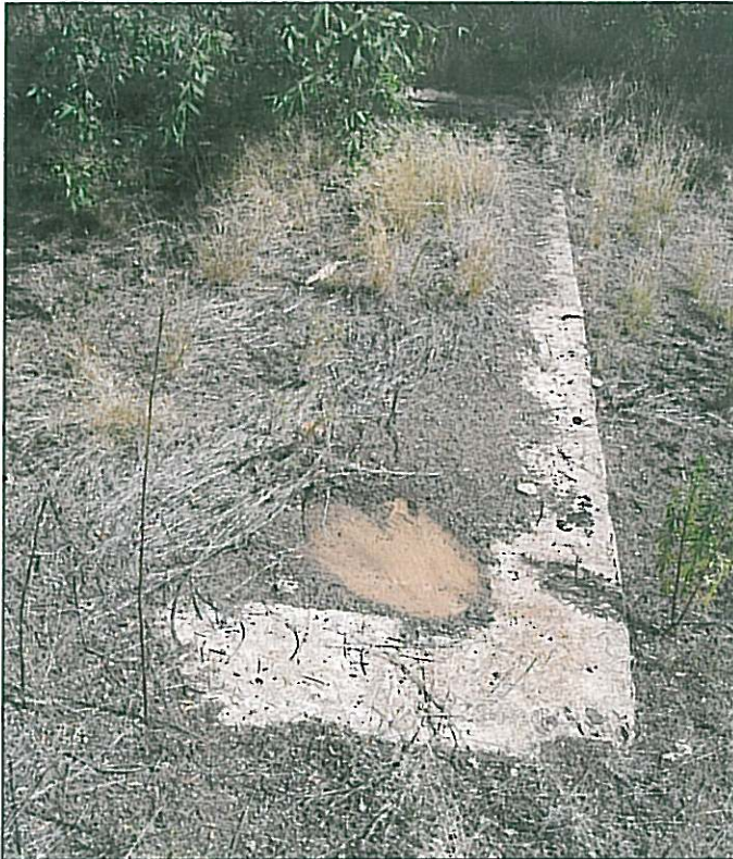
Fig.56 Rim of a concrete floor of unknown origin.
