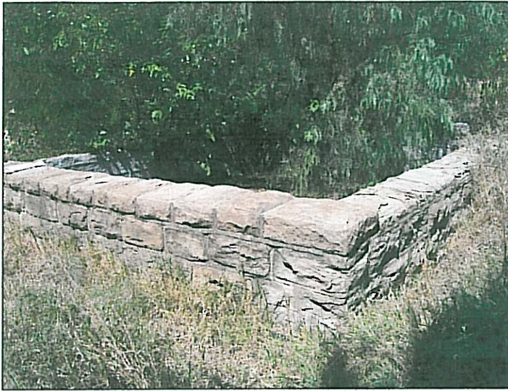
Fig.14 Reservoir dam 1, allegedly built during the time of Pres. Reitz (1889-1895).
