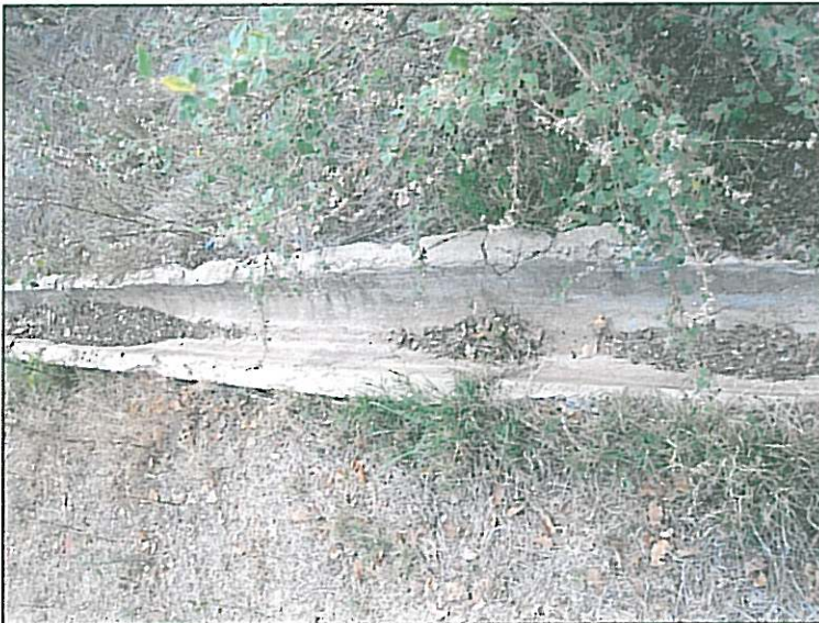
Fig.55 Concrete irrigation furrow.
