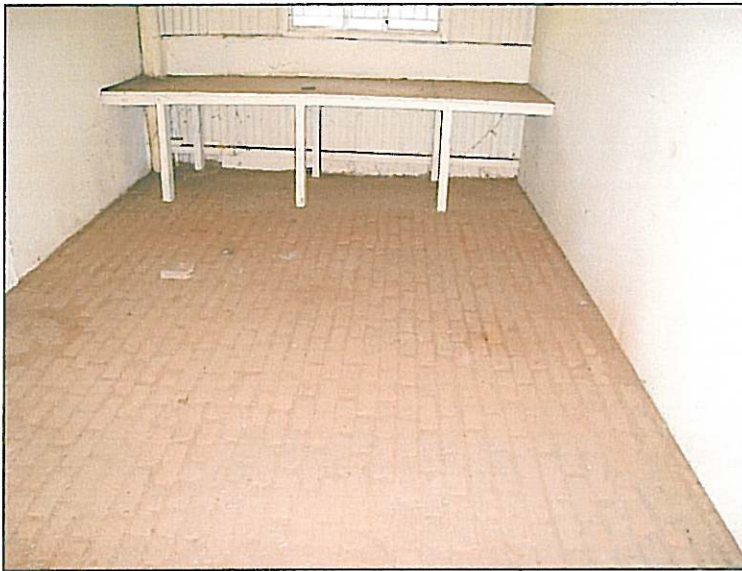
Fig.44 The original brick paved floor of the shed is still intact.
