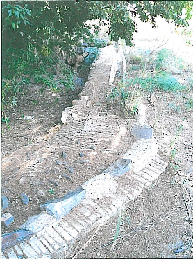
Fig.54 Concrete paving and irrigation furrow.
