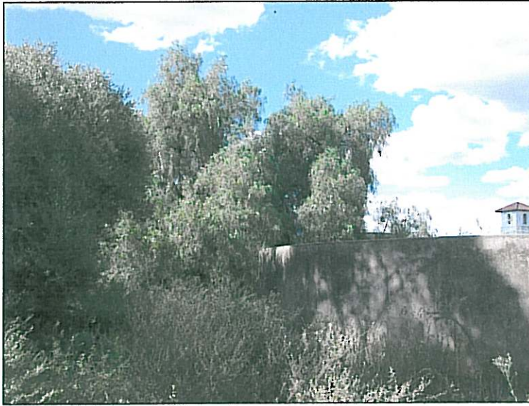
Fig.18 Point C near the water reservoir dam.
