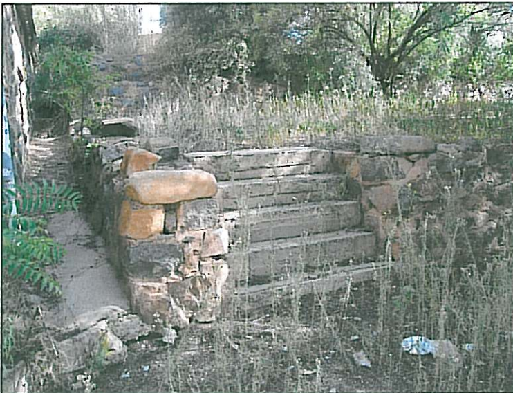
Fig.45 Concrete steps and stone terrace walls behind the kitchen (stables).
