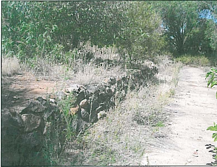
Fig.50 Dolerite terrace wall near large concrete slab.
