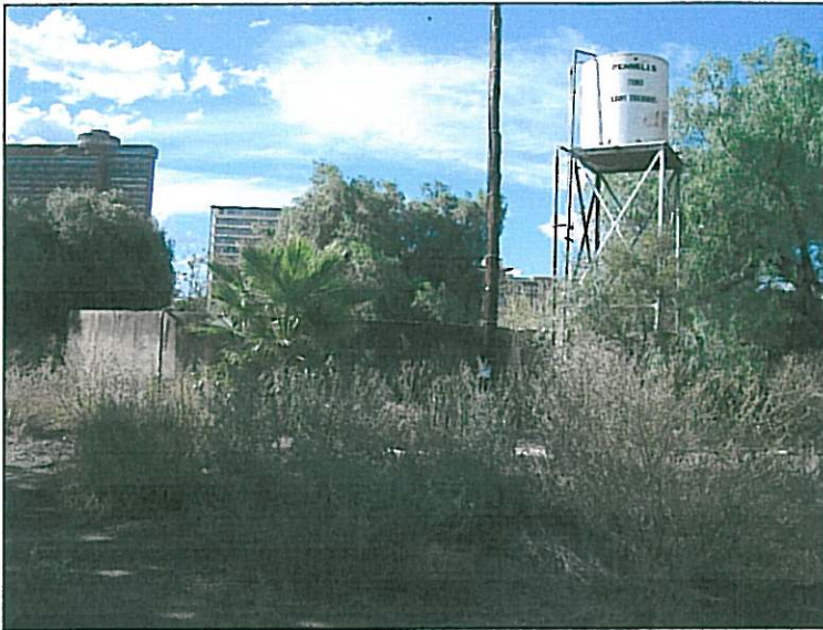
Fig.36 Water reservoir dam 2 and tank installation at the borehole.
