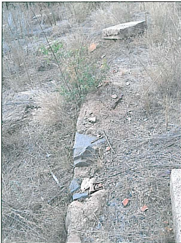
Fig.49 Dolerite terrace steps in back yard.
