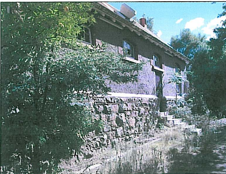
Fig.11 North wall with kitchen back entrance.
