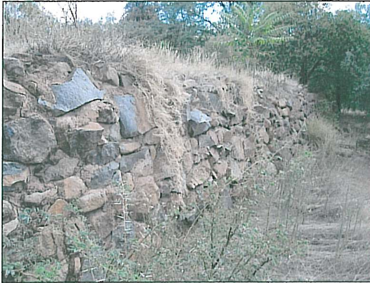
Fig.46 A very prominent stone terrace wall behind the stables
